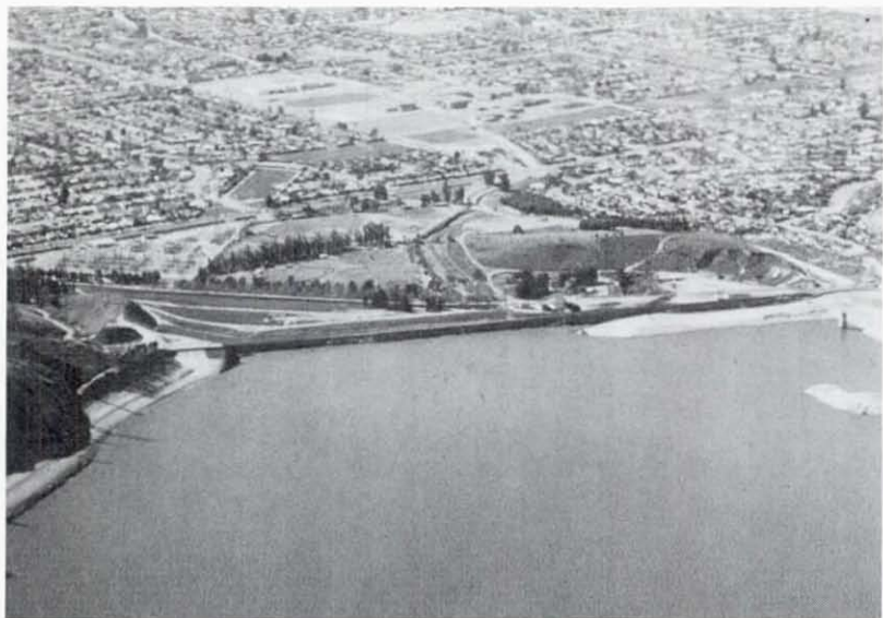
This photograph of the Lower San Fernando Dam, taken a week after the 1971 earthquake, shows the extensive residential area below the dam. Eighty thousand residents were evacuated for three days until the reservoir was lowered to a safe level.
