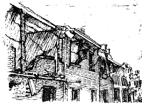
Figure 9 North elevation of bldg.No.2 after the earthquake
