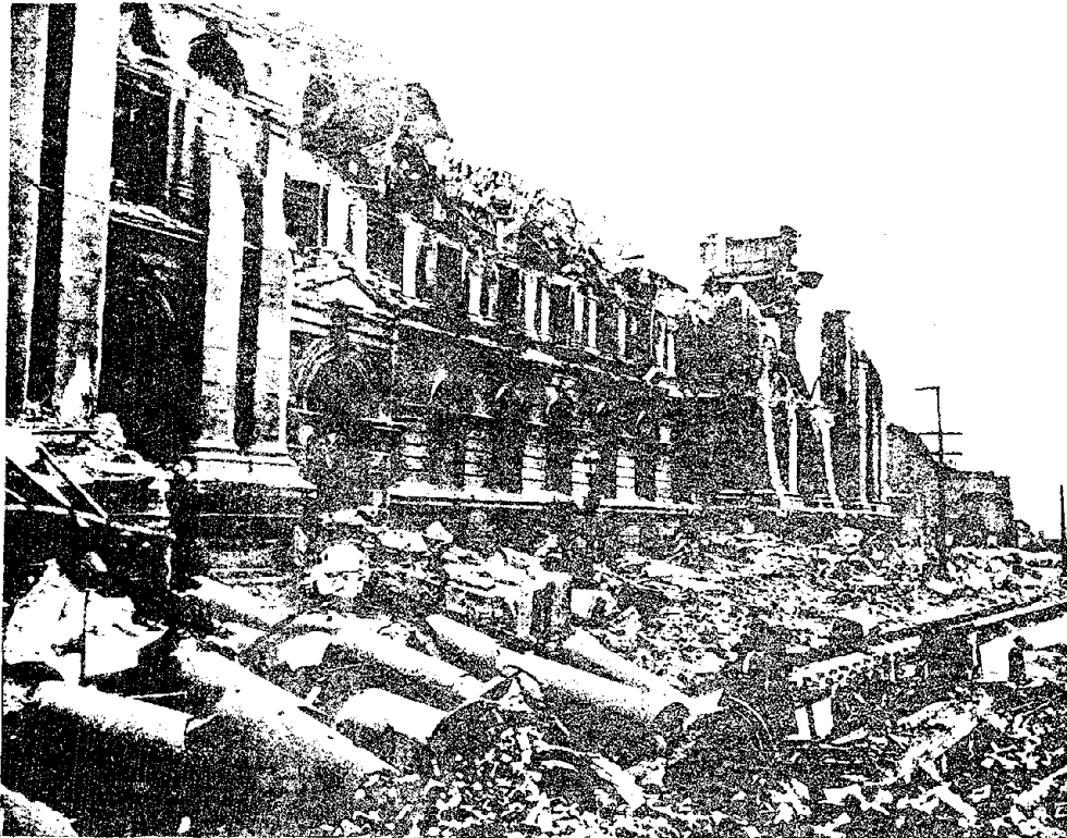
Figures 19a and 19b. San Francisco City Hall, after the 1906 Earthquake.
