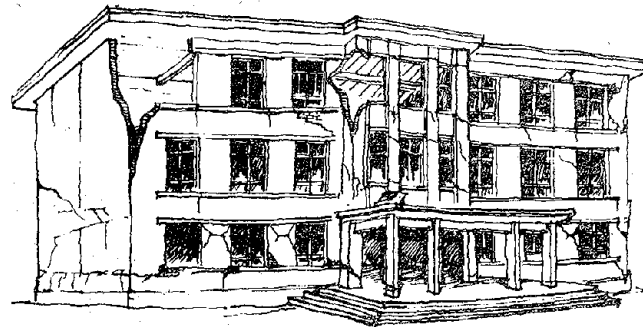
Figure 23 Damaged elevation of classroom bldg. of DXZ primary school
