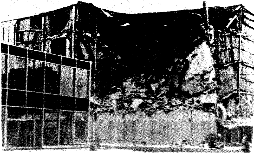
Figure 7 Damage to the J.C. Penney Store, Anchorage, Alaska Note undamaged glass faced building in foreground.
