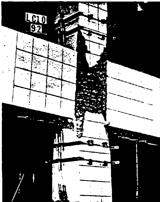
(c) Joint Damaged
