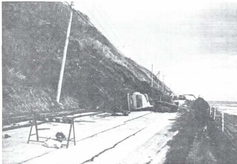
Photo. 2 Damage to Slope along National Highway Route 235, at Irifune Area, Shizunai Town, A Wagon was Buried under Soils.
