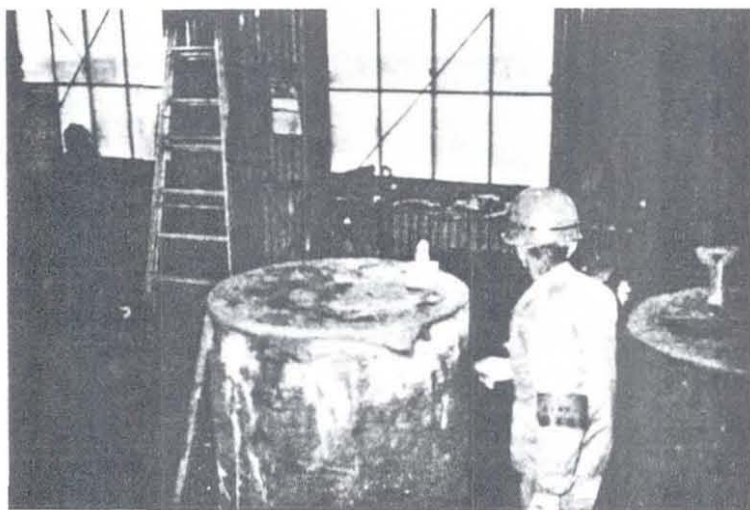
Photo-5. Mortar Casting
