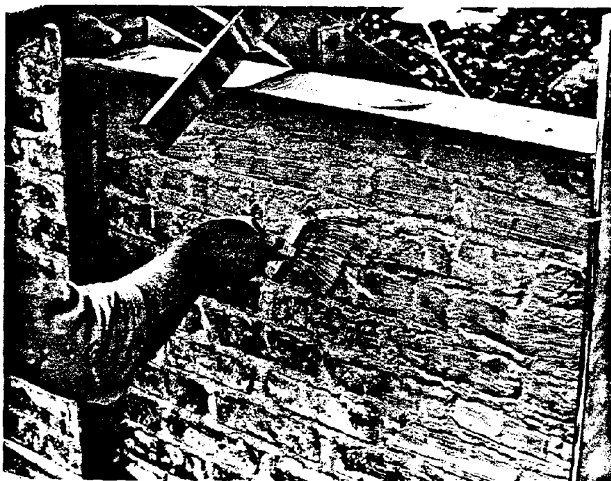
Figure 2.2.10 Brushing Epoxy onto the Surface of the Brick.
