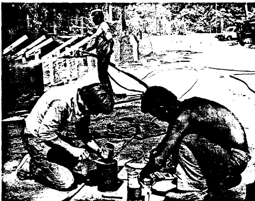
Figure 2.2.9 Mixing Epoxy for Surface Application.
