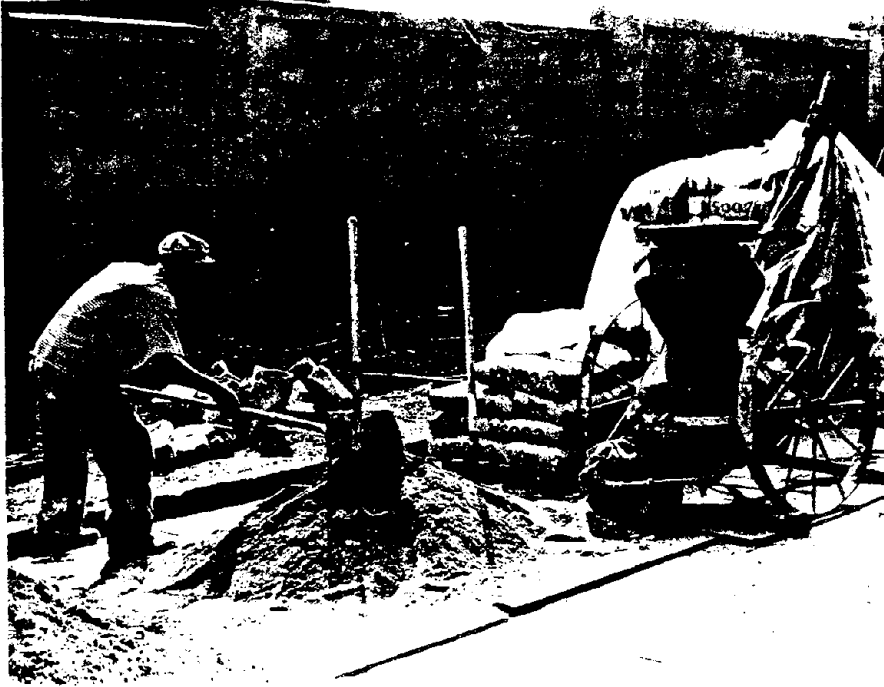
Figure 2.2.4 Mixing the Dry Portions of the Shotcrete.
