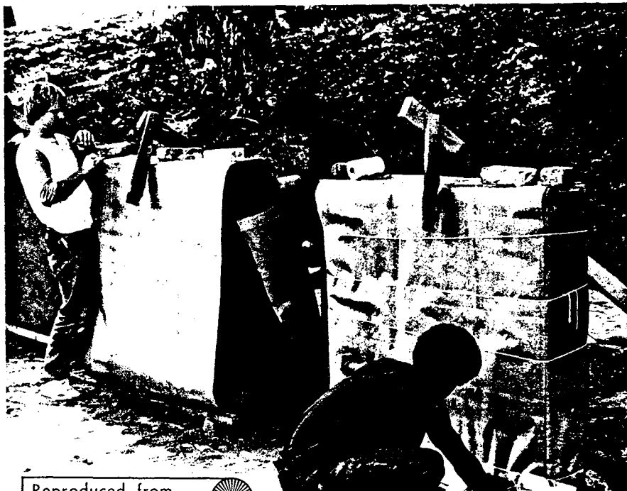
Figure B.67 Covering Specimens with Moisture Barrier.
