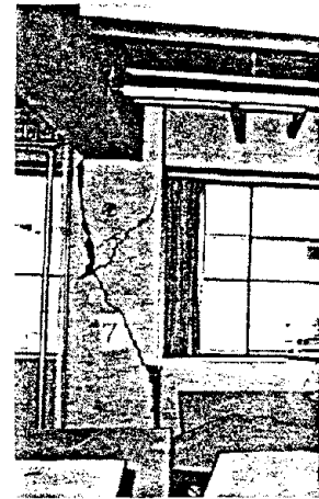
(c) Damage to a Column ( June, 1978)
