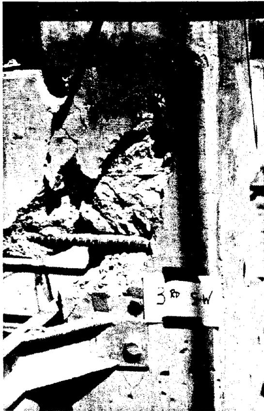
FIGURE 7 DAMAGE FROM THE 1974 TEST AT THE SOUTHWEST CORNER OF THE THIRD FLOOR OF THE ORIGINAL STRUCTURE
