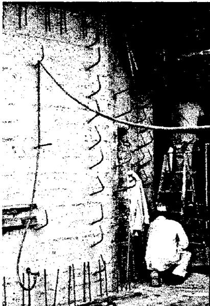
Figure 2 - New rebar dowels epoxy cemented into drilled holes. Vertical bars at floor extend through floor to level below. Randomly spaced hooked bars are to provide additional shear resistance of existing and new section.
