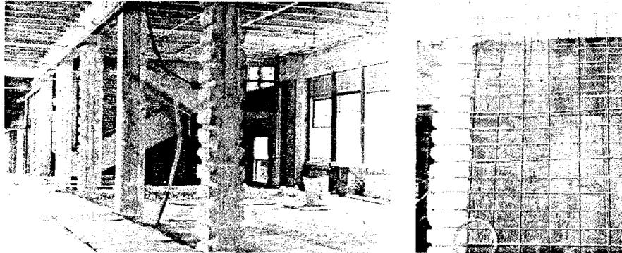
Figure 1 - Notching of existing columns to allow reinforcing for new infill shear walls to bypass. At wall termini, new steel is wrapped around existing column and returned into new construction.
