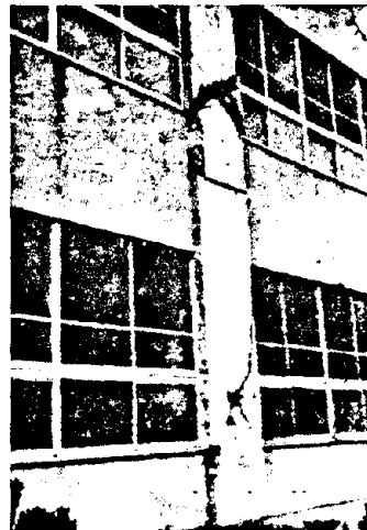
Photo 17. Tonan High School Shearing Destruction of Columns
