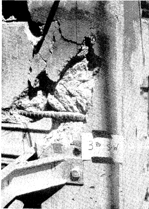
FIGURE 12 DAMAGE FROM THE 1974 TEST AT THE SOUTHWEST CORNER OF THE THIRD FLOOR OF THE ORIGINAL STRUCTURE
