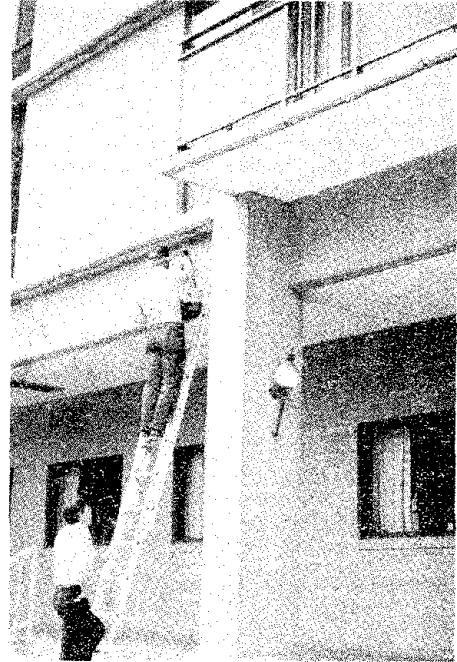
Figure 3 - Locating Reinforcement by Pachometer
