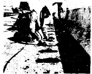
(e) Grouting blockouts
