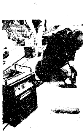
(c) Stud welded through blockouts in slab
