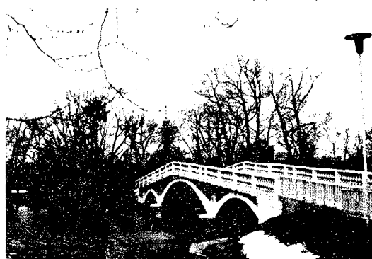
Fig. 5 An open spandrel arch bridge
