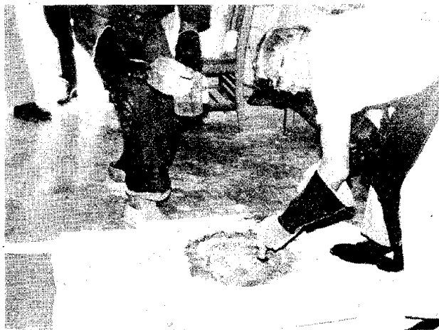
Fig. III The tack coat being applied to the pothole.
