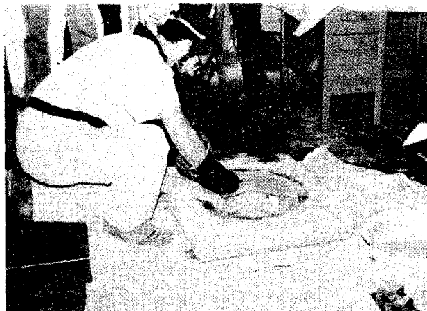
Fig. V Leveling of the mix after placing.
