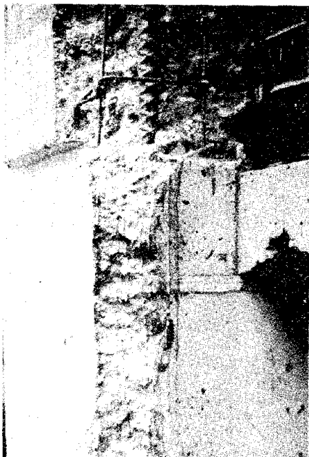
c. Epoxy Coating on Reinforcement to Eliminate Continued Chloride Attack
