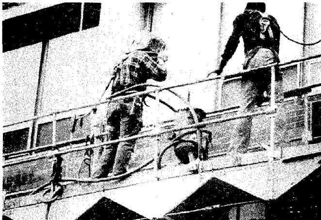
b. Cleaning by Sand Blasting
