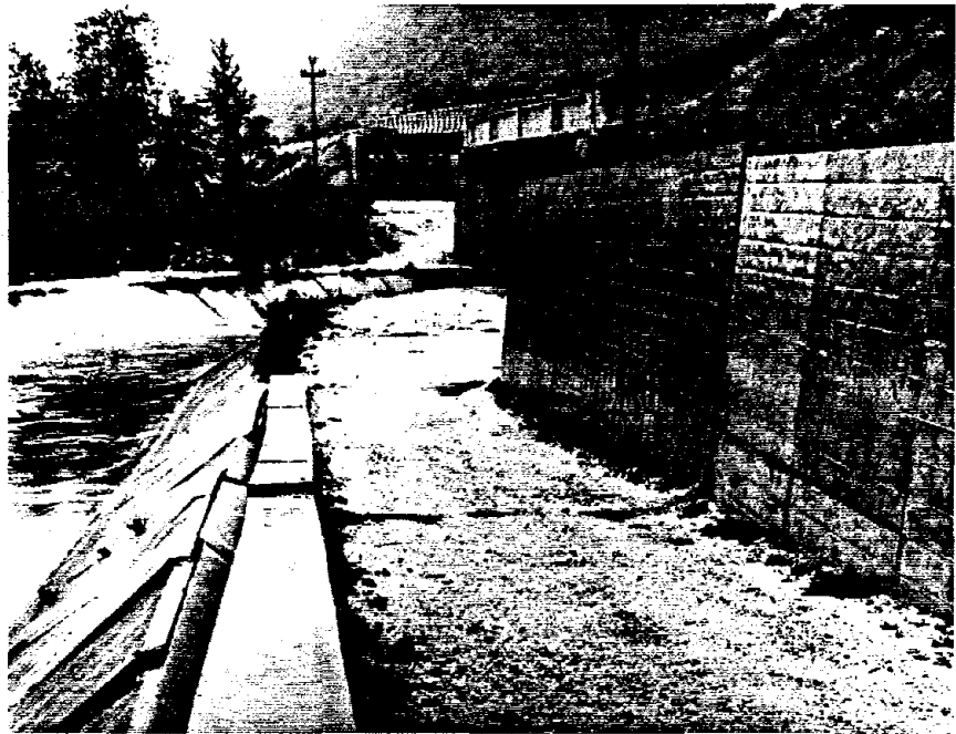
FIGURE 1.29 - DAMAGE TO EMBANKMENT RETAINING WALL AND CANAL, UDINE-CARNIA-TARVISIO HIGHWAY - FROM (10)
