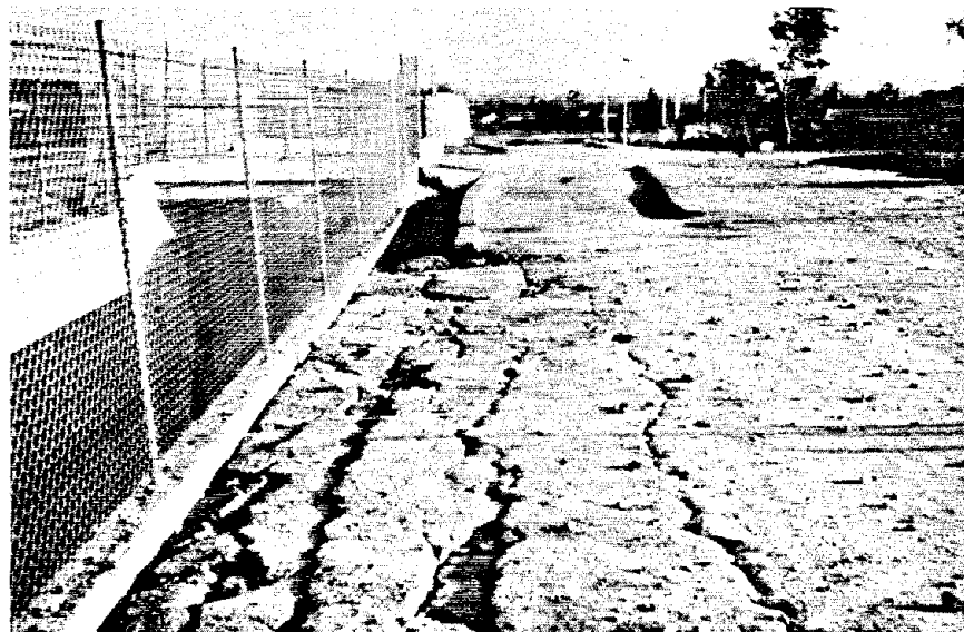
FIGURE 1.25 - WILSON CANYON CHANNEL:CRACKING IN SOIL AS A RESULT OF WALL DISPLACEMENT - FROM (67)
