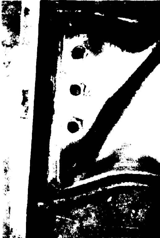
Fig. 4.25 Photo of Distorted Bolt Holes of Specimen 22.
