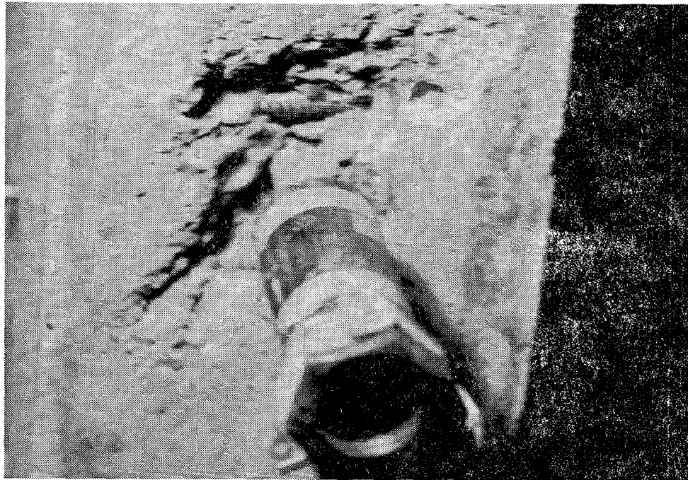
(a) PHOTO OF SPECIMEN AFTER BREAK OUT OF CONCRETE CONE.
