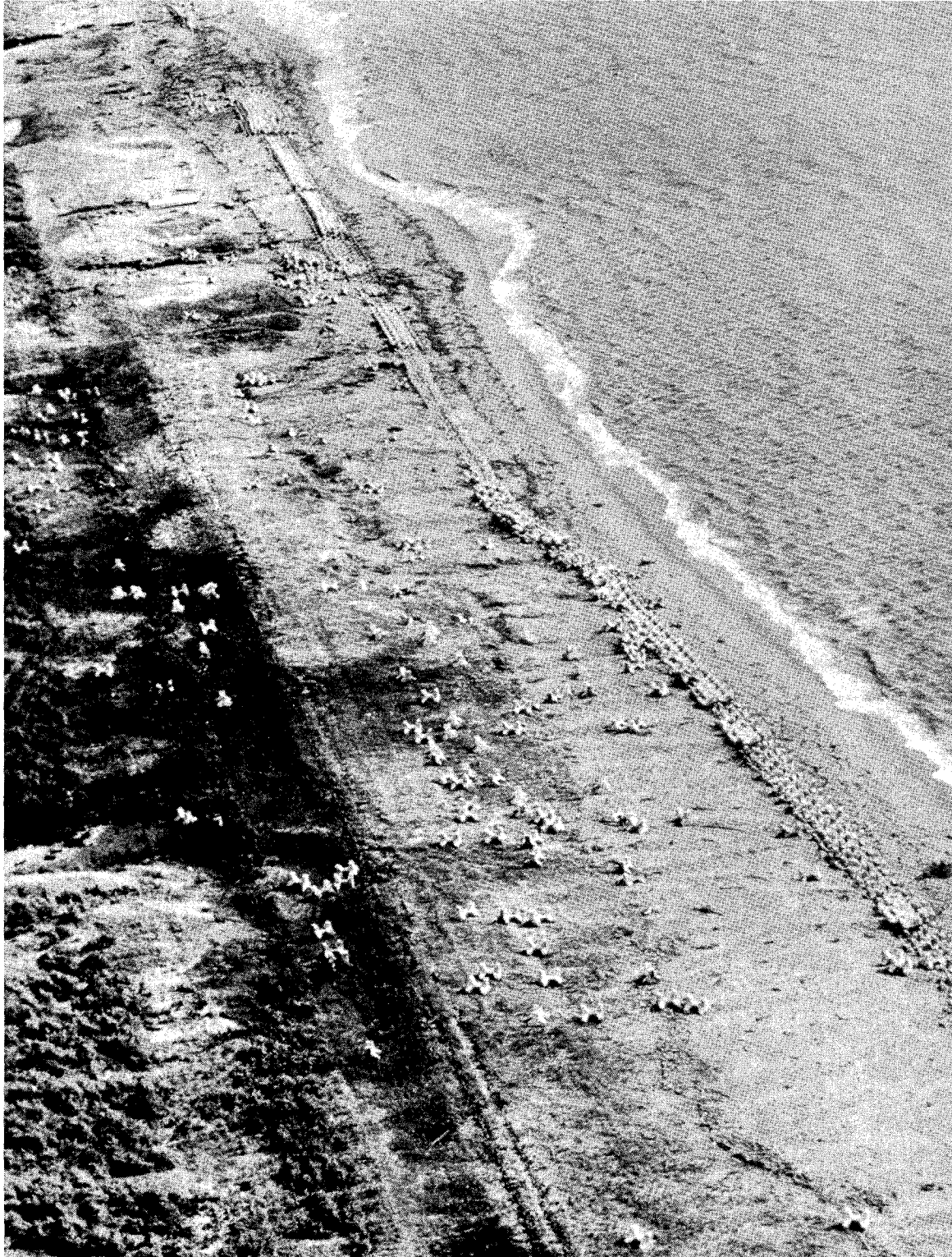
FIGURE 17 Protective concrete units weighing 4 metric tons were scattered by the tsunami at Mizusawa Beach near Minehama Village in Akita Prefecture. Source: Akitakai Newspaper Publishing Company, 1983.
