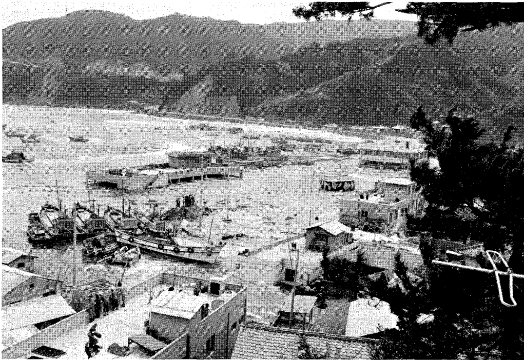
FIGURE 16B Damage to floating structures in Imweon, Korea. Source: Korea Maritime and Port Administration.
