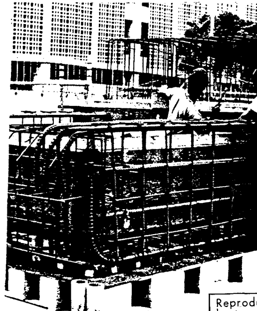
Fig. 4 - Reinforcement for Box Girder Hinge Component
