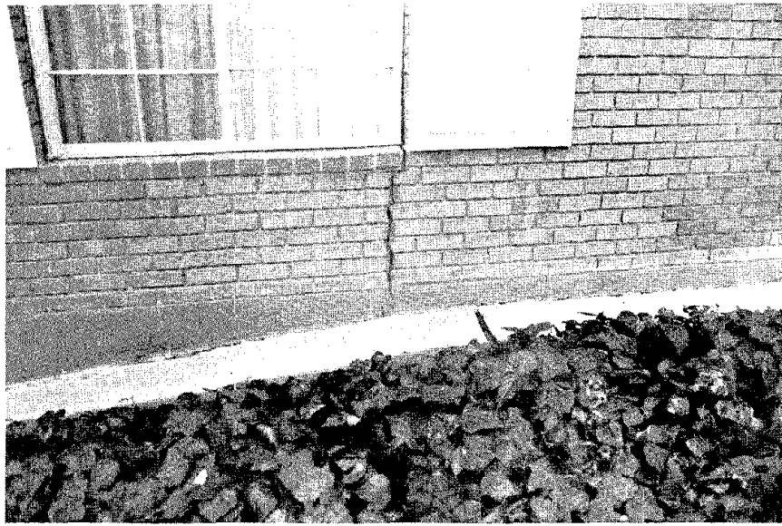
FIGURE III-10 DAMAGE DUE TO SURFACE FAULT RUPTURE IN CONTRA COSTA COUNTY
