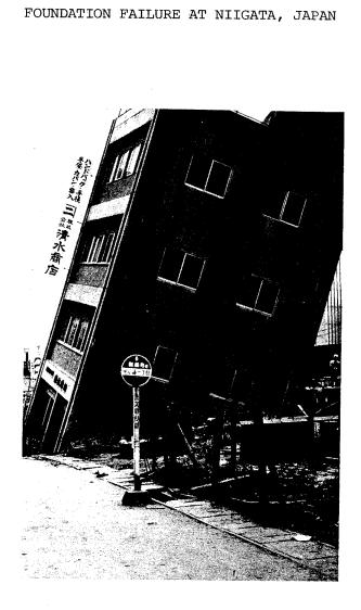
SOURCE: Seed, H. Bolton, and Kenneth L. Lee, "Liquefaction of Saturated Sands During Cyclic Loading," Journal of the Soil Mechanics and Foundations Division, American Society of Civil Engineers, November 1966, p. 106.
