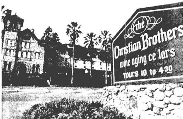
A structural report indicated that Greystone could not withstand a moderate earthquake
