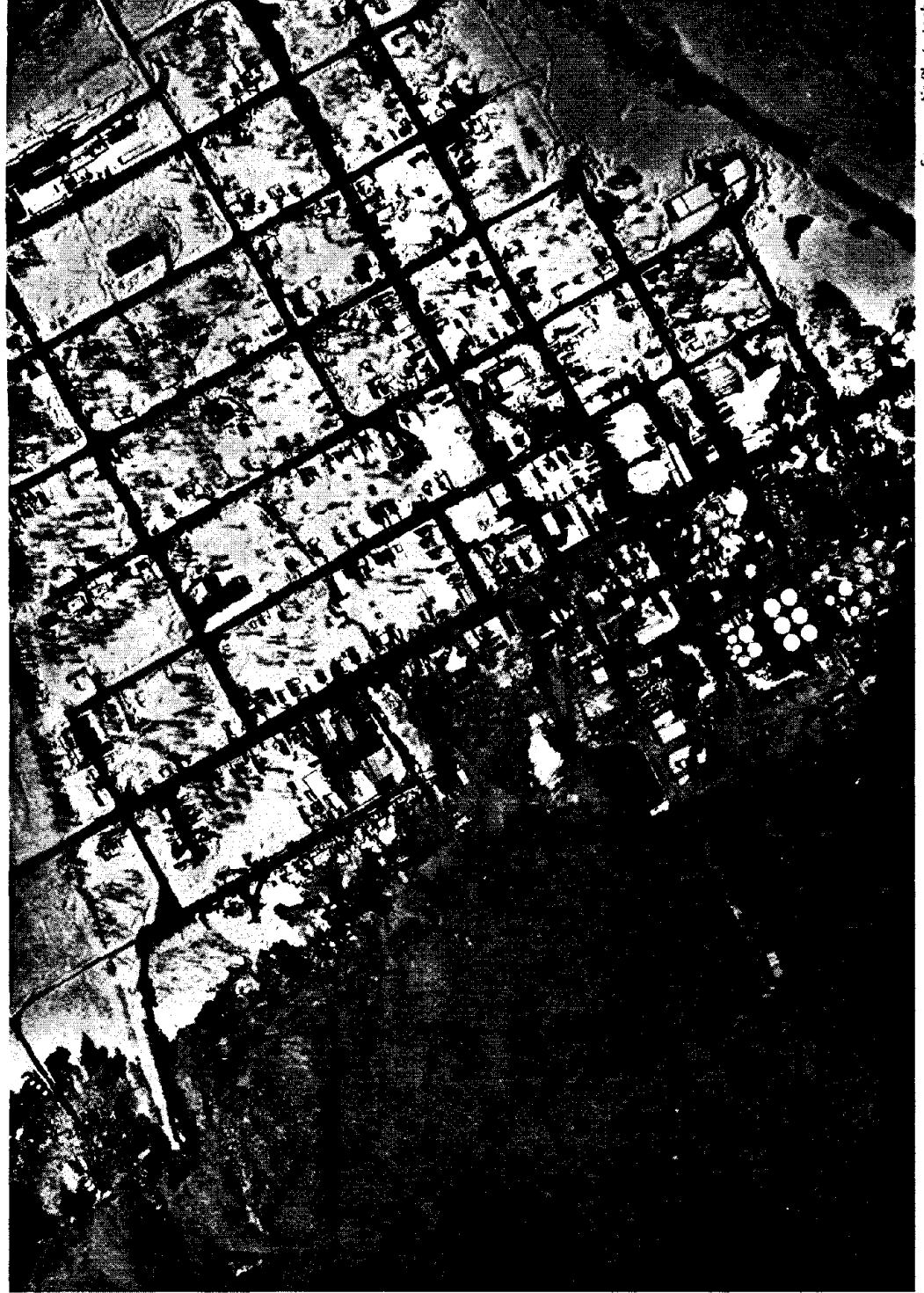
Figure 18. Damaged Old Valdez
