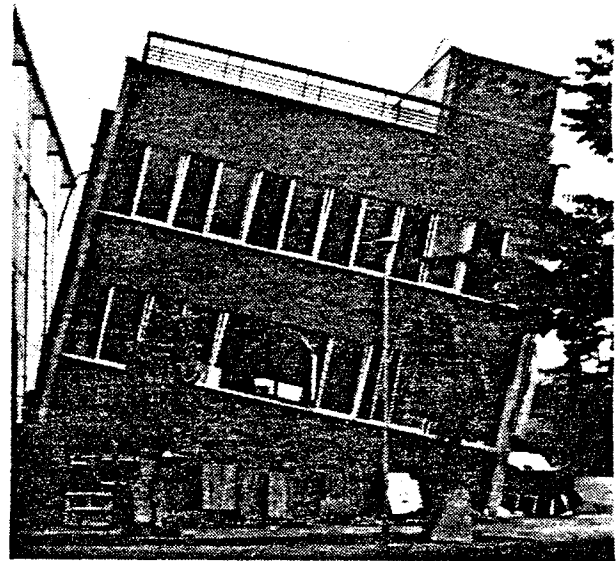
Fig. 2 Torsional effects
