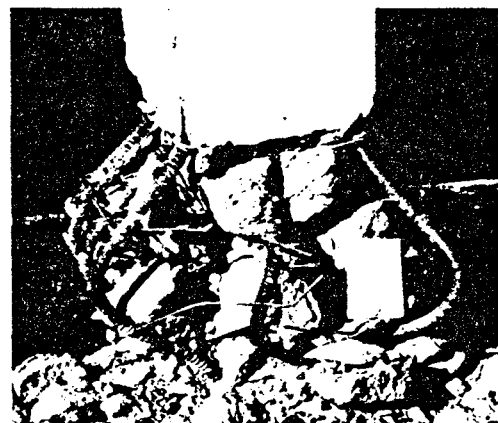
Fig. 4 Detail of Column G4 Failure
