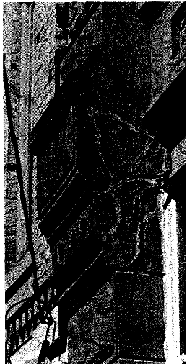
Fractured Facade Element
