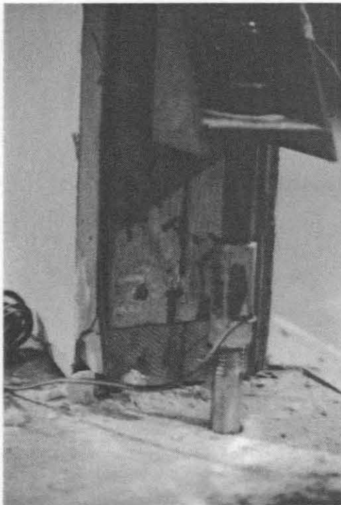
Figure 46: Specimen PD-4 Run No. 2 Splitting Failure of Bottom Sill-Plate and End Stud Test No. A-11, Frequency = 0.5 Hz Peak Command Displacement = \pm 2.8 Inches
