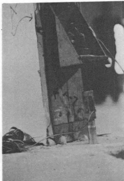
Figure 44: Specimen PD-4 Run No. 2 Splitting Failure of Bottom Sill-Plate and Edge-Stud Test No. A-10, A-11, Frequency = 0.5 Hz Peak Command Displacement = \pm 2\text{-}1/2 Inches, \pm 2.8 Inches
