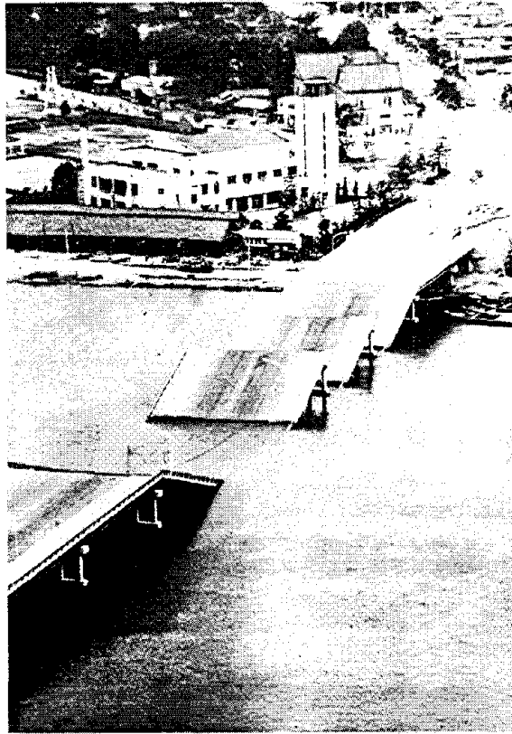
FIGURE 2-3 Failure of the Showa Bridge during the 1964 Niigata earthquake. Source: Seed and Idriss (1967).
