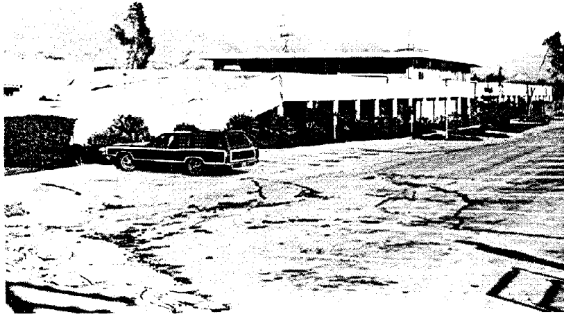
FIGURE 2-5 Damage to the San Fernando Juvenile Hall facility during the 1971 San Fernando earthquake. This building partially collapsed when soils under the foundation liquefied. Even though the building is on a relatively flat slope, uneven displacements occurred and essentially pulled the building apart. Note the surface cracks in the parking lot in the foreground. Photograph: Courtesy of G. W. Housner.
