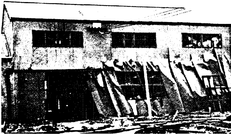
FIGURE 2-9 Building pulled apart by lateral spreading during the 1964 Niigata earthquake. Source: Kawasumi (1968).
