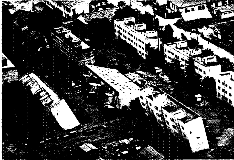
FIGURE 2-1 Tilting and settlement of apartment buildings in Niigata, Japan, because of liquefaction of the underlying soil during the 1964 Niigata earthquake. Photograph: Courtesy of G. W. Housner.
