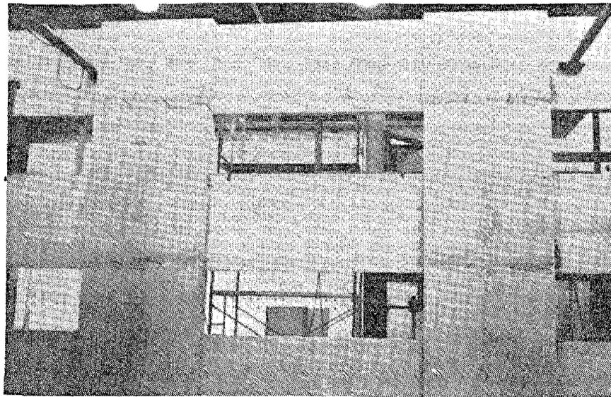
Fig. 2.35 The completed R/C pier strengthening scheme
