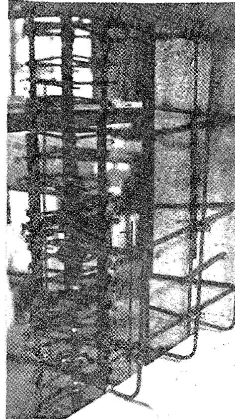
Fig. 2.31 Hooked #3 longitudinal bars in window area
