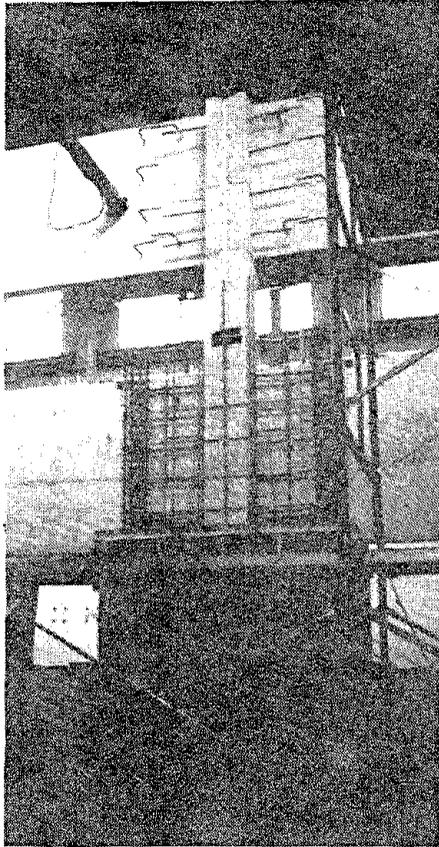
Fig. 2.34 Exterior formwork for casting stage 1
