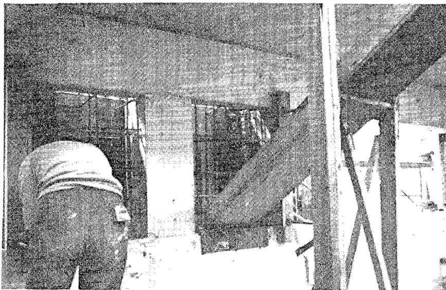
Fig. 2.32 Concrete was placed from the interior of the frame using a chute which emptied into the formwork
