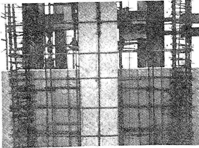
Fig. 2.30 Transverse and longitudinal steel in place
