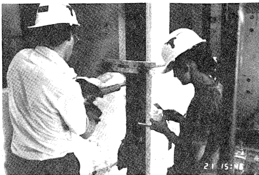
Fig. 3.23 Epoxy application procedure
