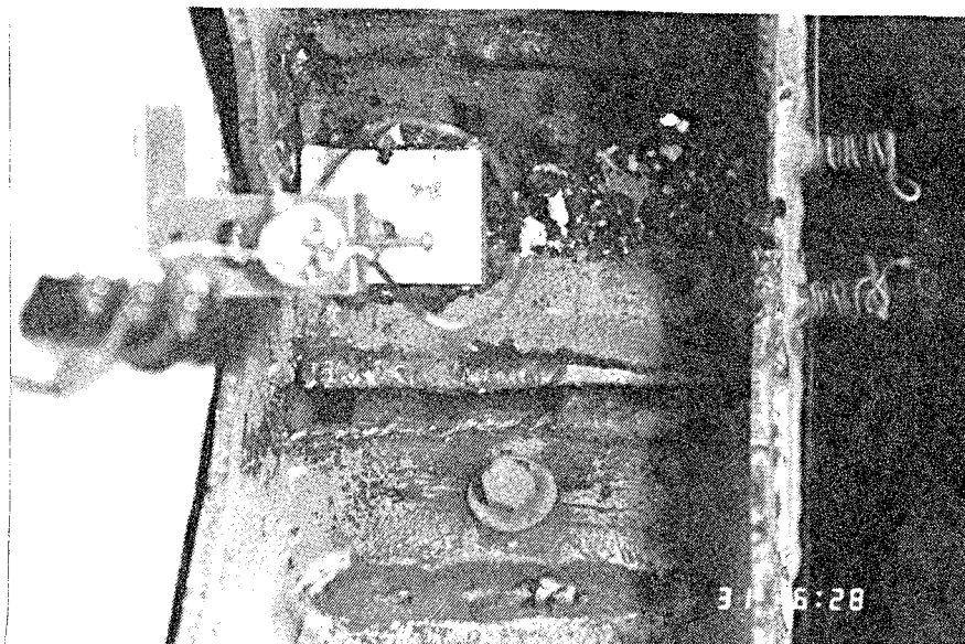
Fig. 4.14 Weld failure at bottom of brace T2
