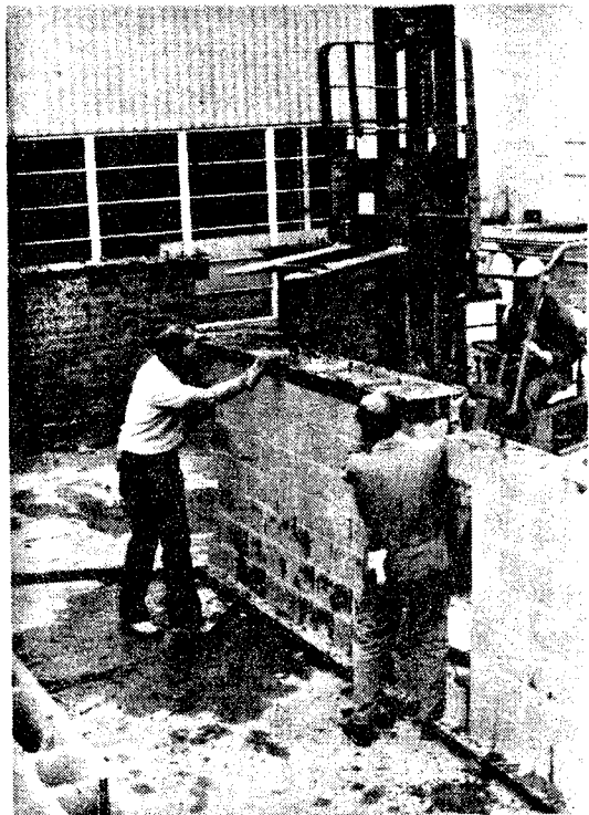
FIG. 2.3 CONSTRUCTION OF TEST SPECIMEN
