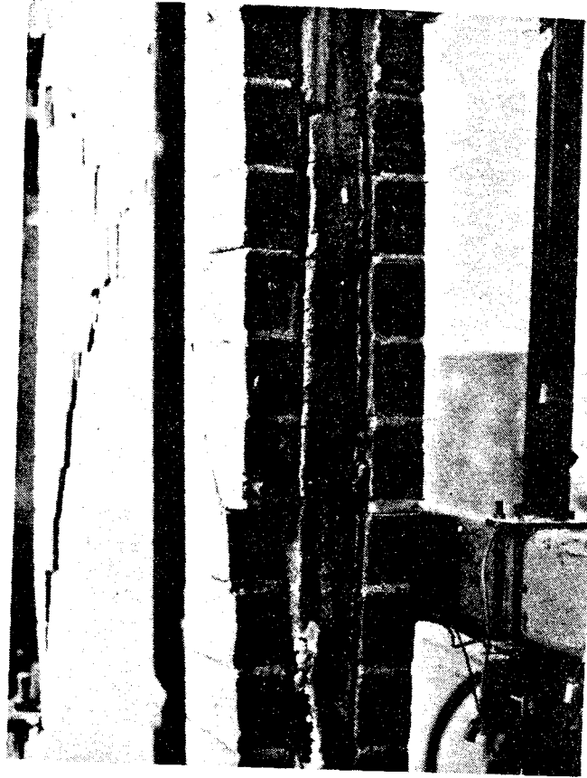
FIG. 4.2 CORE SPLIT IN GROUTED CORE BRICK WALLS
