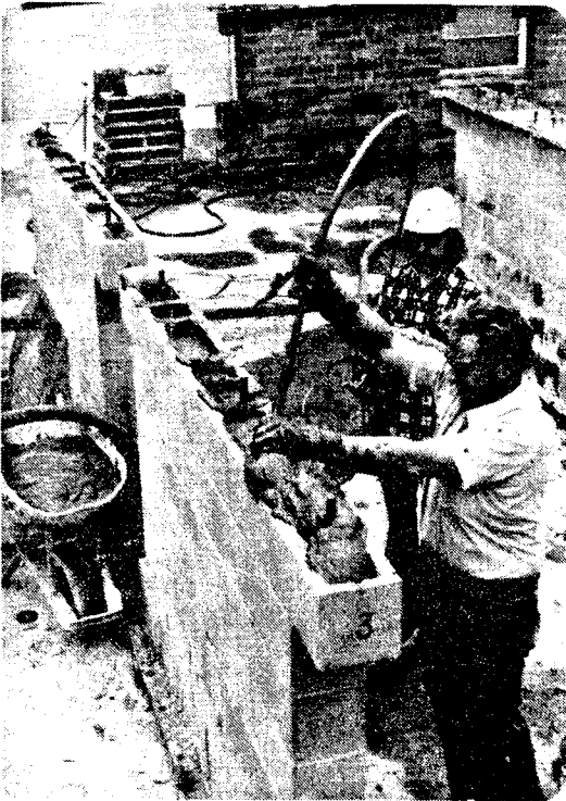
FIG. 2.3 CONSTRUCTION OF TEST SPECIMEN
