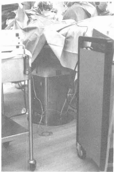
Figure 5.48 Base of an operating table. Tables are not always built-in as in this example.
