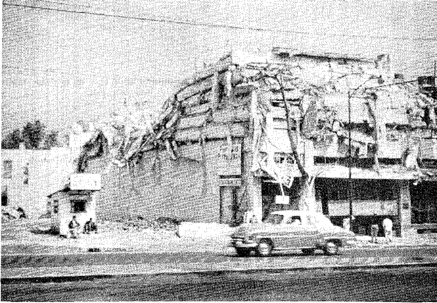
FIGURE 11 Collapse of an eight-story building in Mexico City in 1957. Such collapses, in which the floors are stacked like a deck of cards, have been observed in several earthquakes. The epicenter of the 1957 Mexico earthquake was 200 miles south of Mexico City. Similar collapses occurred during the September 19, 1985 Mexico earthquake. Buildings that were not designed to resist earthquakes are especially susceptible to damage from distant events. (Photo provided by George W. Housner)
