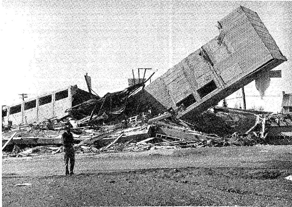
FIGURE 9 This six-story, reinforced-concrete apartment building vibrated strongly before collapsing during the 1964 Alaska earthquake. It was newly built in Anchorage and was a lift-slab type, relying on the two vertical elevator/stair shafts to provide earthquake resistance. There were no recording instruments in or near the building. (Photo by George W. Housner)
