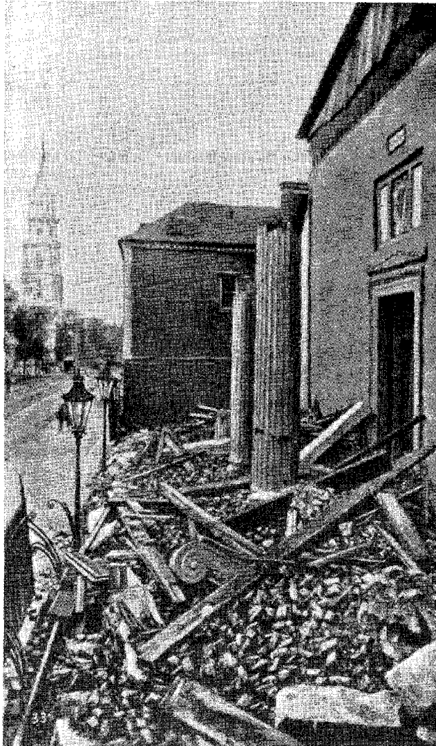
FIGURE 2 Photograph of building collapse in Charleston, South Carolina. This destructive earthquake occurred August 31, 1886 and caused considerable damage. Its estimated magnitude was 7.7. Source: Dutton (1890).
