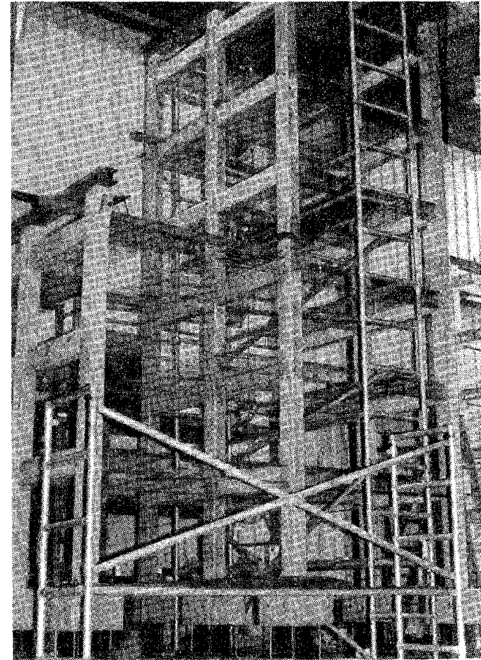
Figure 3.3 Short-Direction Frames on Steel Foundation. (Before Casting the Long-Direction Frames).
