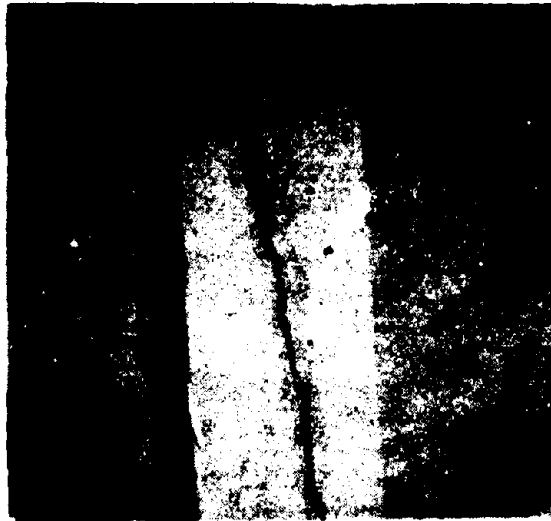
CRACK ALONG THE BEAM
