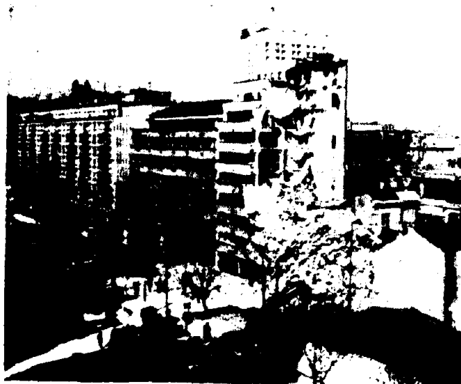
Fig.2 "Casata" building (noted "A" in fig.1) after collapse at the March, 4 th 1977 Vrancea Earthquake.
