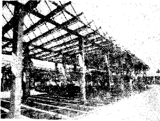
FIG. 1 Collecting instalation for solar energy, for 1200 places at Alfa, Beta and Gama hotels in Saturn resort. The place of the collector being on auto parking roof.
