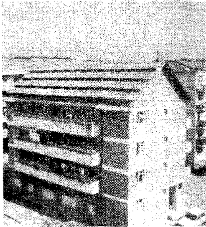
FIG.10 Solar installation for the domestic warm water preparation at Valenii de Munte, for 8 apartaments using propylen glycol as an antifreeze solution.
