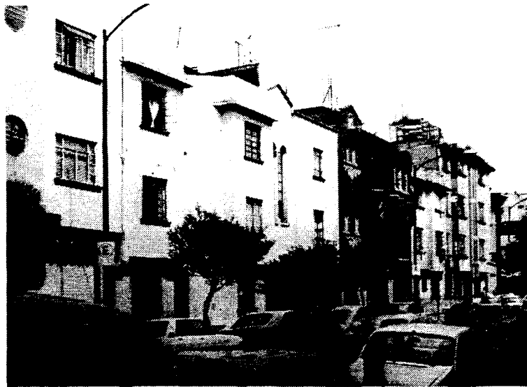
Figure 3. Low-rise residential structures in downtown Mexico City.
