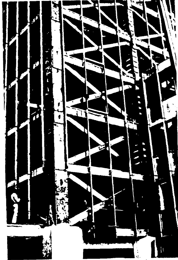
FIGURE 6 Post-Earthquake Repair of Damaged Building
