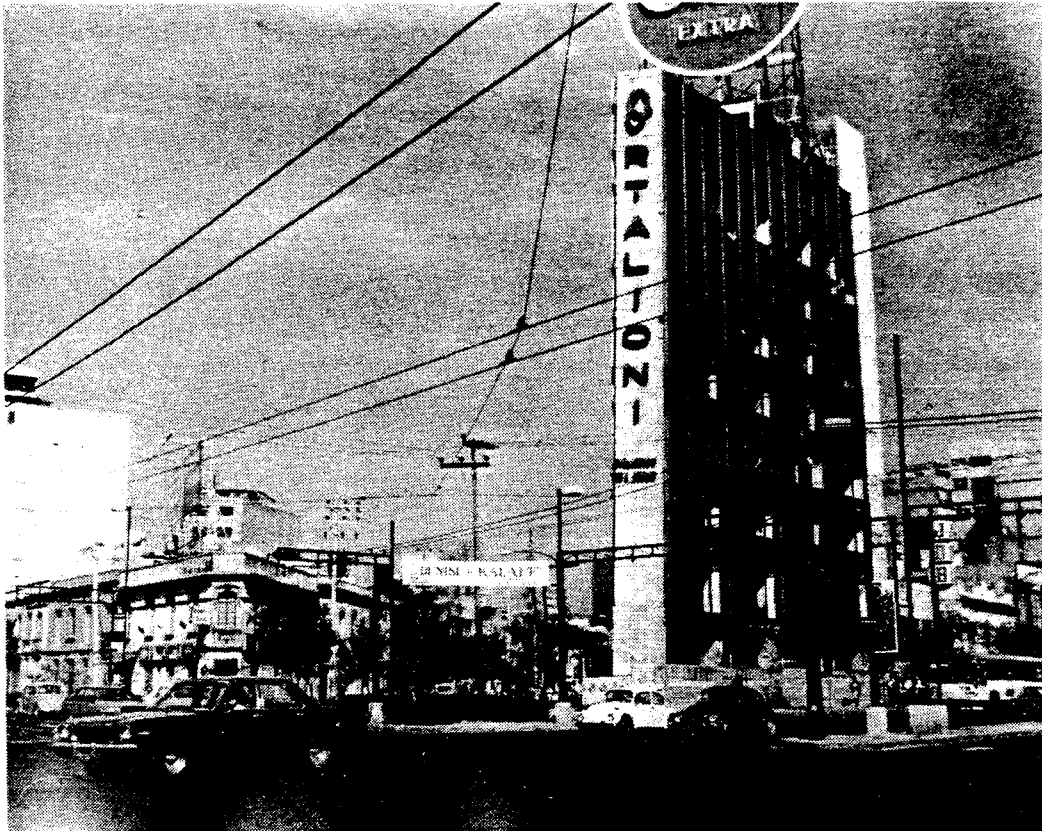
Figure 11. Distortion of a wedge shape building at a corner. This building was later demolished.
