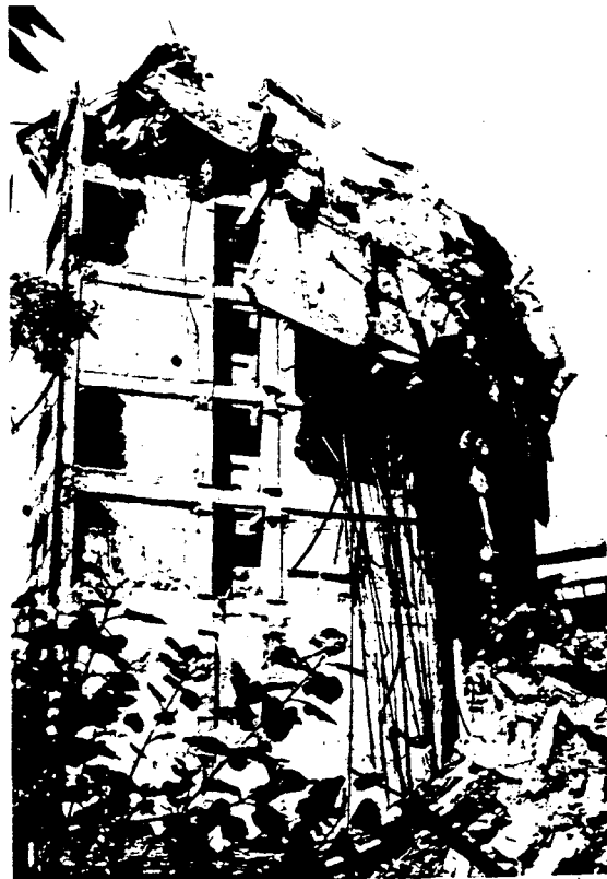
FIGURE 3 Collapsed Upper Floors, Reinforced Concrete High-Rise Building
