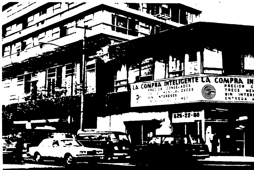
Example of Pounding Damage Between Adjoining Buildings
