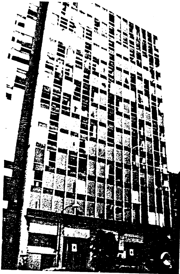
The larger glass panels tended to experience the more serious glass damage.
