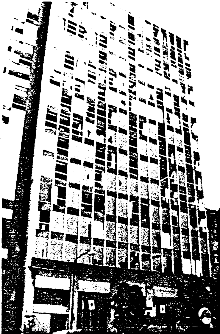
Metal frame glazing systems tended to receive higher amounts of serious glass damage than the more rigid systems.
