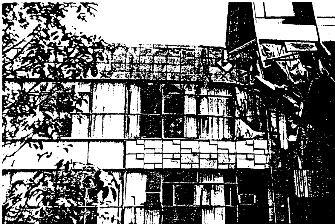
Buildings with partial height adjoining buildings experienced higher amounts of serious glass damage through pounding.
