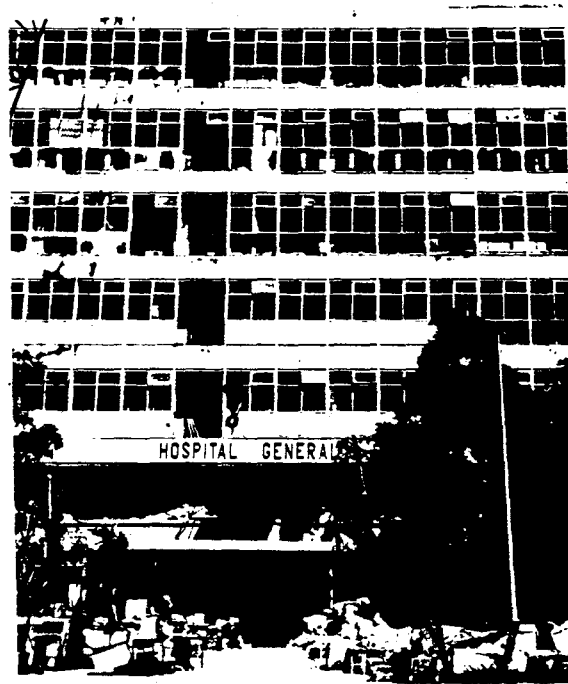
FIGURE 9 Damaged Window Wall Assembly
