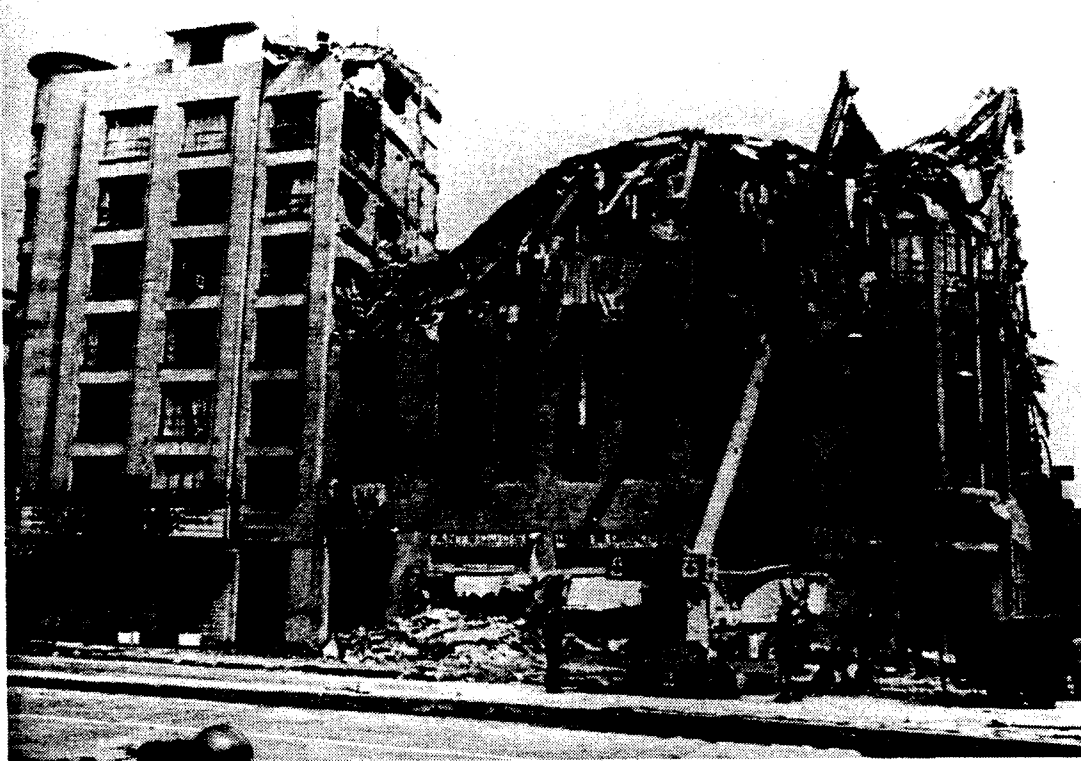
Figure 6. Upper story failure.
