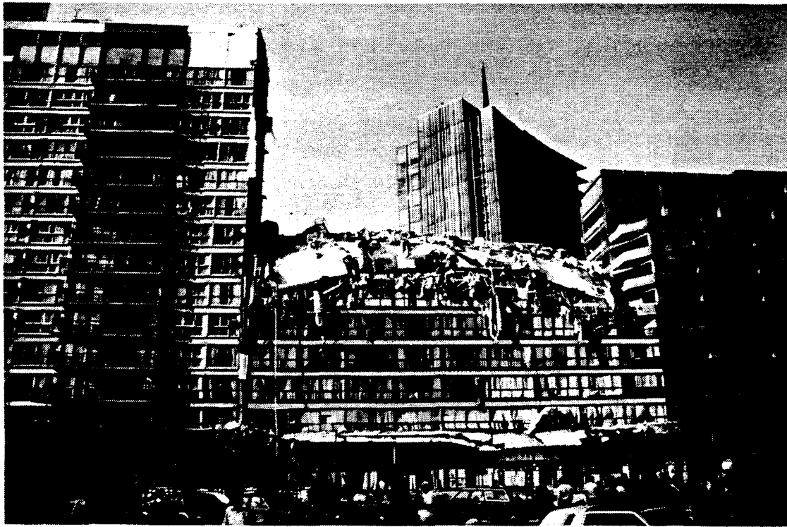
Figure 7. Mid-story failure.
