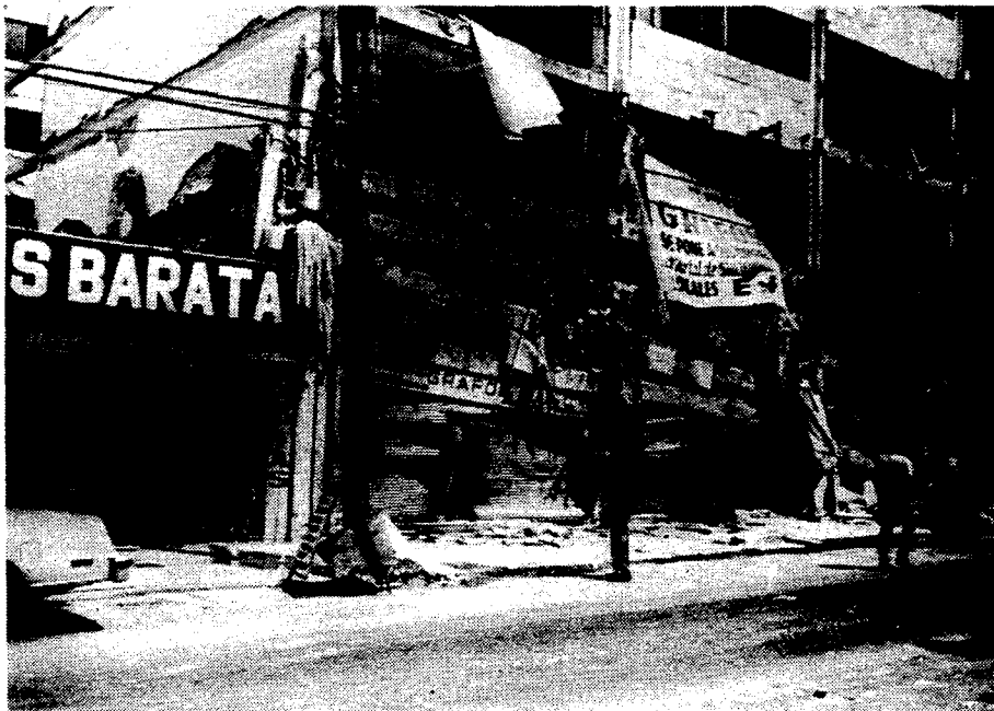
Figure 9. Weak first floor failure
