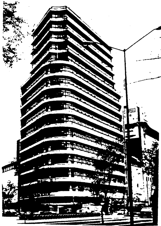
Abandoned Flat Iron Building After Earthquake Still Unoccupied in February 1987
