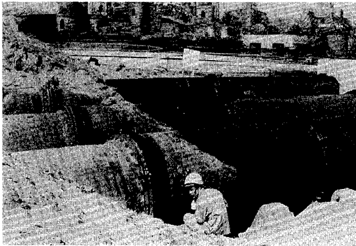
Photo 6 Pull-out and Dislocation at Joint of Tail Race Pipes in Area ⑧
