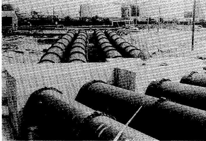
Photo 5 Horizontal Movement of Tail Race Pipes in Area ⑦ (On-ground Pipes)
