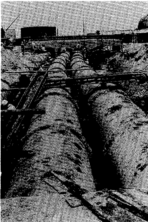
Photo 3 Horizontal Movement of Tail Race Pipes in Area ⑤
