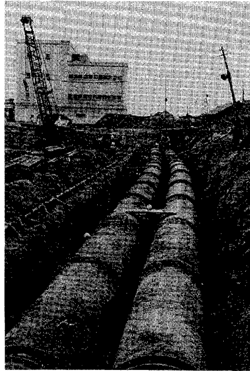
Photo 2 Horizontal Movement of Head Race Pipes in Area ②
