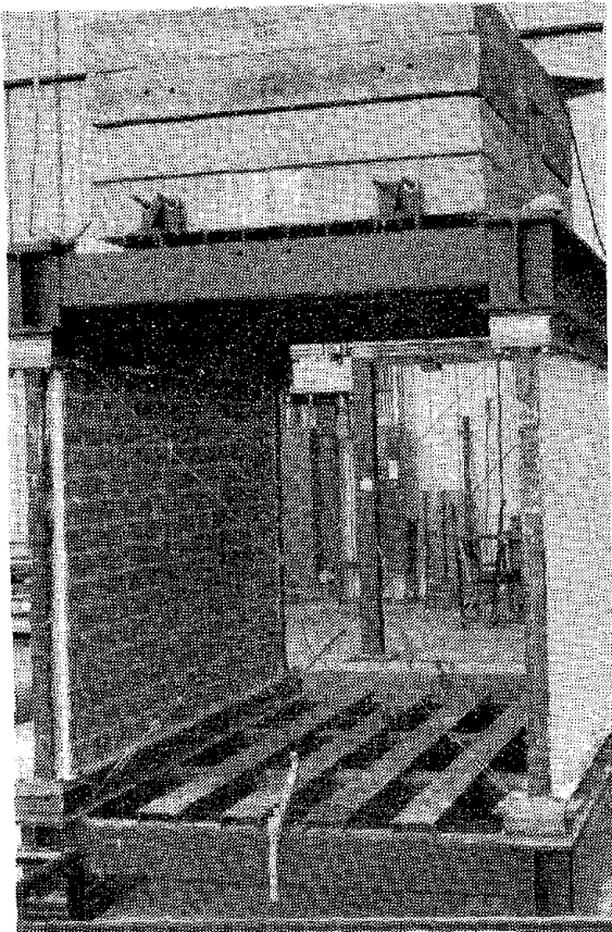
Figure 12: Masonry Partition within the Frame Ready for Dynamic Loading
