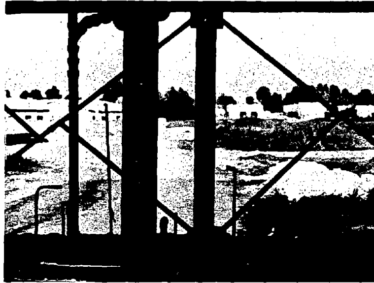
Figure 3-11 Steel bracing of building in figure 3-10.
