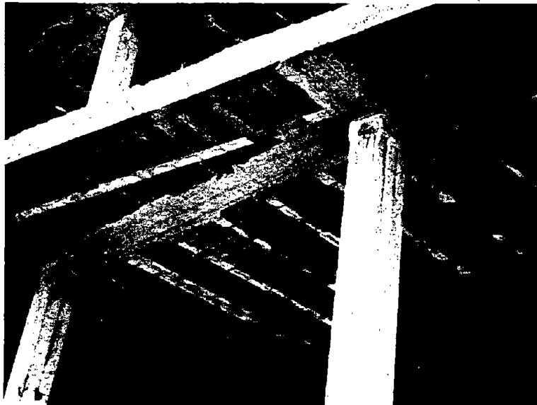
Figure 3-14 Typical concrete frame construction in Iran
