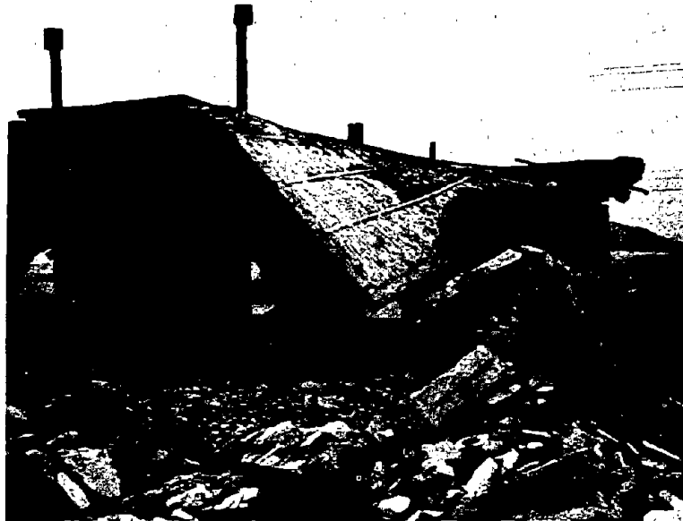
Figure 3-3 Roof collapse in an unreinforced masonry bearing wall structure. The roof is brick infilled steel beam (jack arch) system which is very common in Iran.
