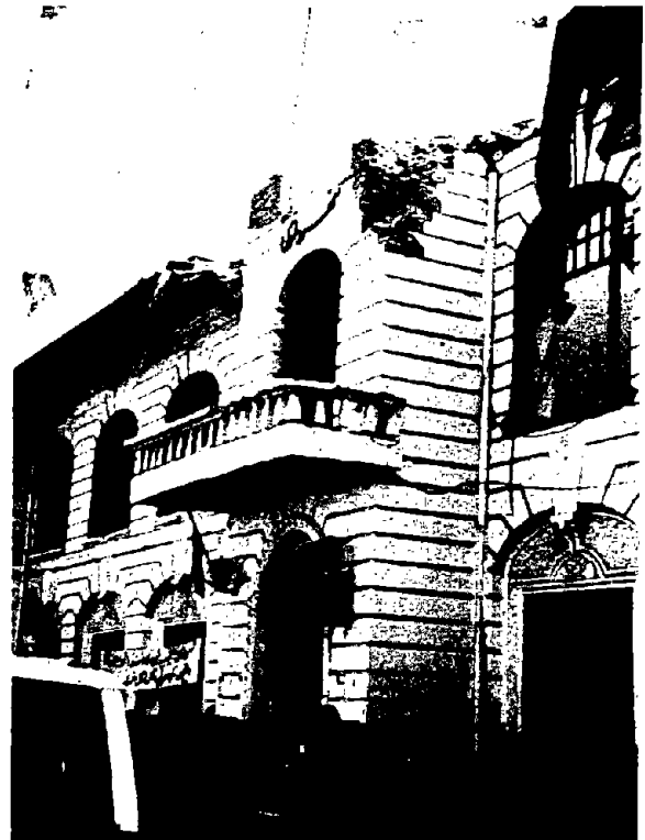
Figure 3-3 Roof collapse in an unreinforced masonry bearing wall structure. The roof is brick infilled steel beam (jack arch) system which is very common in Iran.
