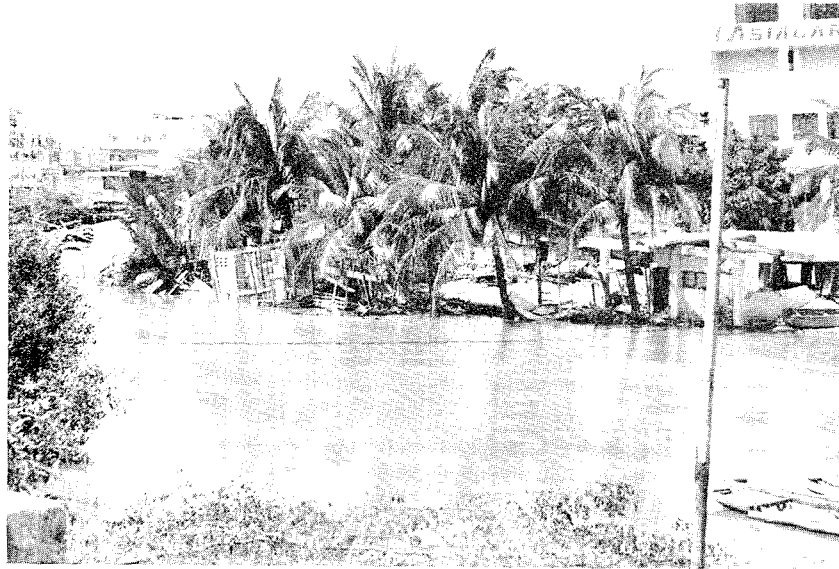
Photo.4 Lateral spreading of the right bank which pushed the wooden house into the river
