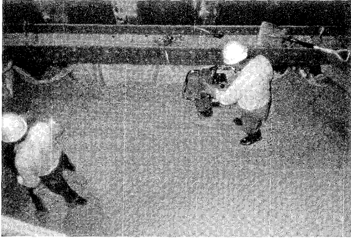
Photo 12 Compacting of gravel
