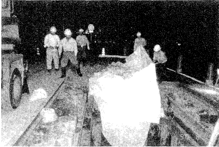
Photo 6 Insertion of filter into excavated hole
