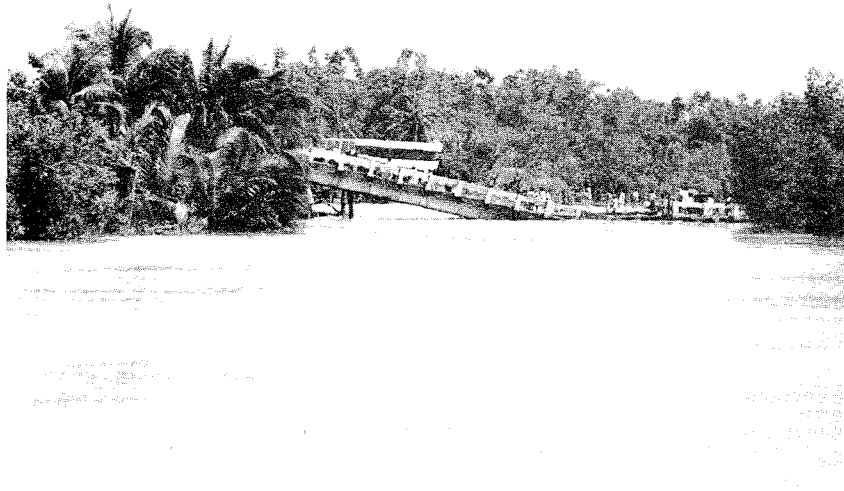
Photo.5 The four-span concrete plate-girder Magsaysay Bridge in Dagupan City collapsed due to lateral spreading of the riverbanks toward the stream channel and/or loss bearing capacity of the piers due to liquefaction
