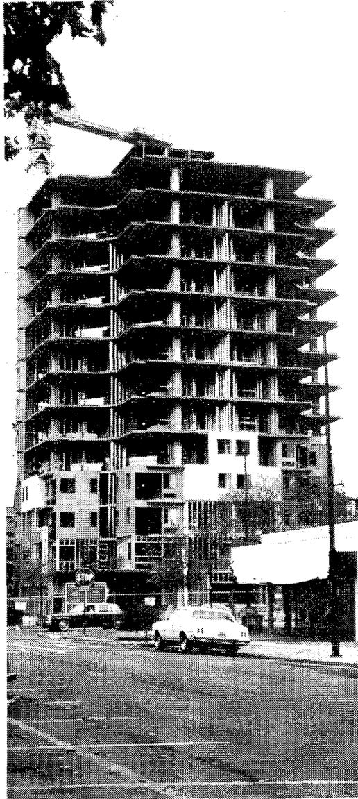
**Fig. 8.1 A Multistory Building With Flat-Slab Construction**
