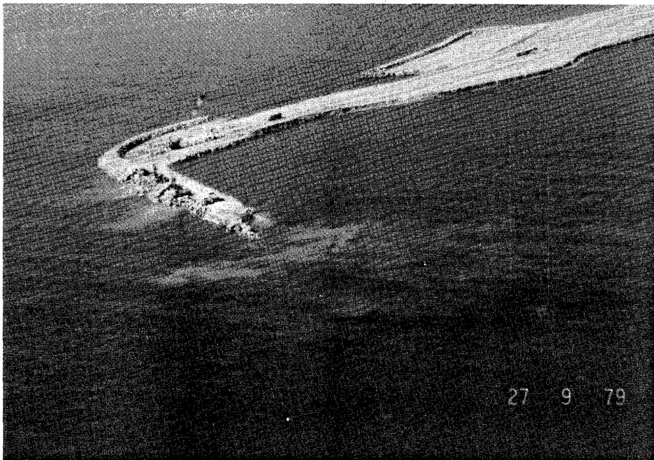
Fig. 3 PORTION OF FILL INVOLVED IN SLIDE OF OCT. 16, 1979
