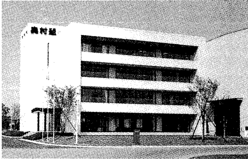
Figure 6 Okumura Company Demonstration Building in Tsukuba Science City
