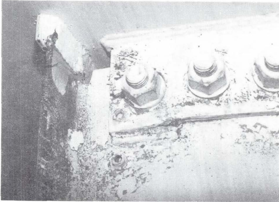
Figure 3.69 Fracture of Bottom Flange and Lower Web Weld (Specimen 13)
