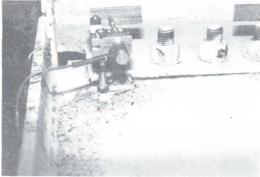
Figure 3.47 Fracture of Top Flange and Upper Web Weld (Specimen 4)
