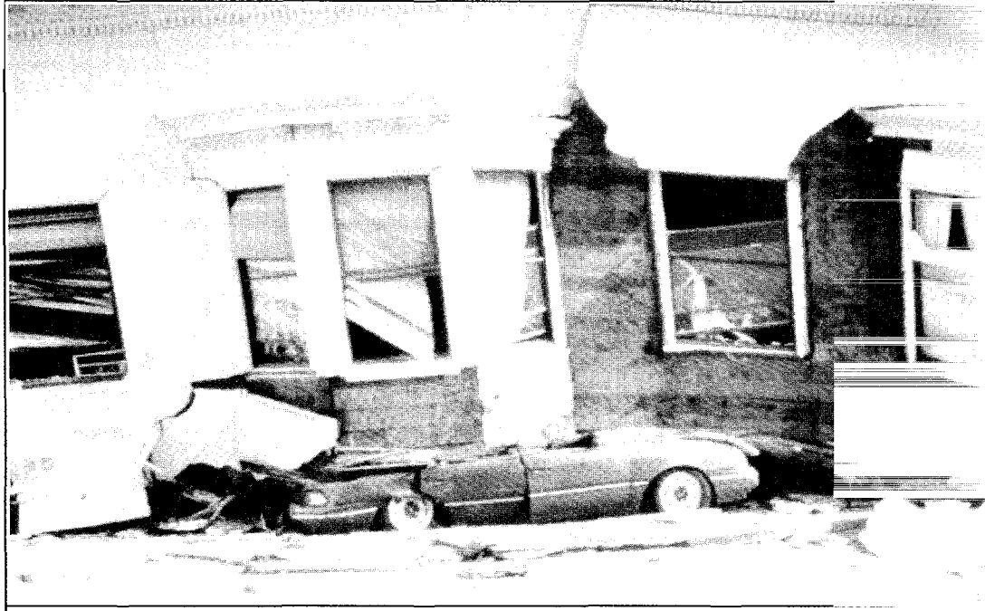
Damage During the Loma Prieta Earthquake
