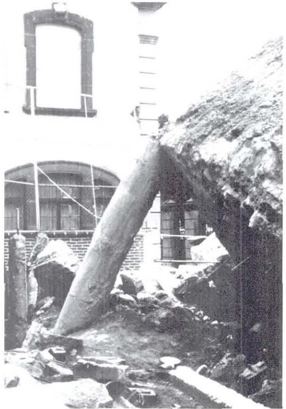
Figure 6: Foundation pile pulled out of ground by toppled building.
