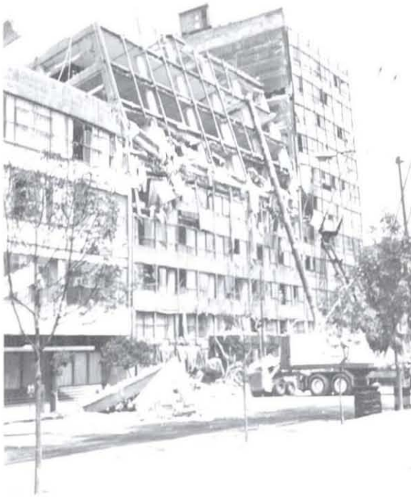
Figure 8. Upper portion of building failed.
