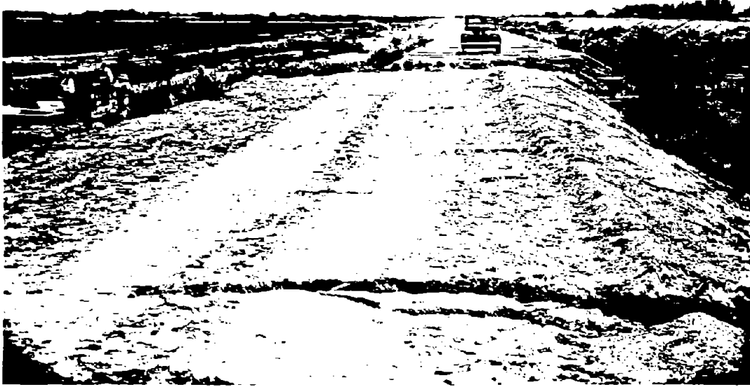
Figure 2-12: CLOSE-UP OF THE FRACTURE ZONE ACROSS THE LEFT ALL-AMERICAN CANAL EMBANKMENT
