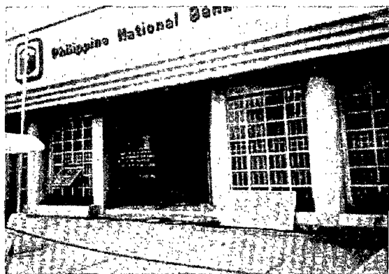
Photo 16. Philippine National Bank looking from Angel Fernandez Avenue. The buildings seems to have settled a little but no damage could be found on the exterior wall.
