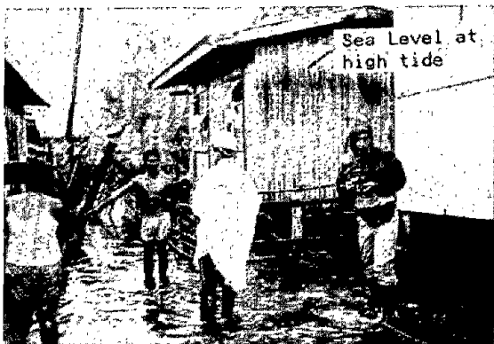
Photo 43. Damage in Barrio Narvacan. Traces of water at high tide are seen on the eaves. (Courtesy of Dr. M. Hakuno).
