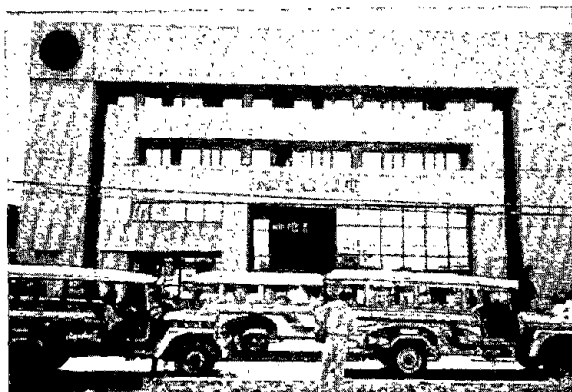
Photo 37. The Insular Life building, one of two buildings constructed with pile foundations in Dagupan City. The building is located in the non-liquefied area. Several small cracks were observed on the non-structural exterior walls and these were caused by ground shaking.
