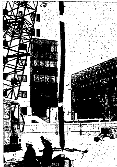
Photo 25 Damaged Pile of the NHK-Building (S. Kawamura et al.) 13
