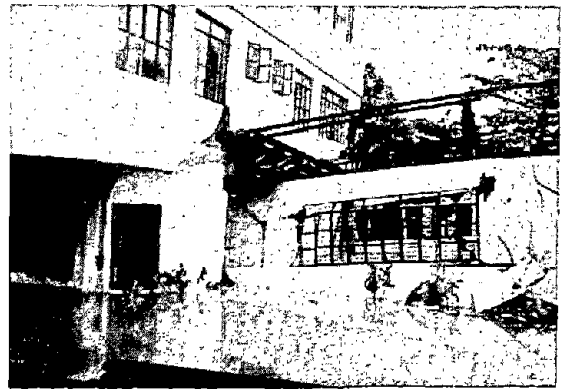
Photo 7. The Asia Career building. The low rise portion was dragged down by the settlement of the high rise portion (Courtesy of Dr. I. Towhata).
