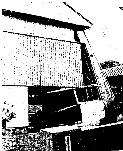
Photo 39 Damage to the School Gymnasium due to Displacement of the Foundations
