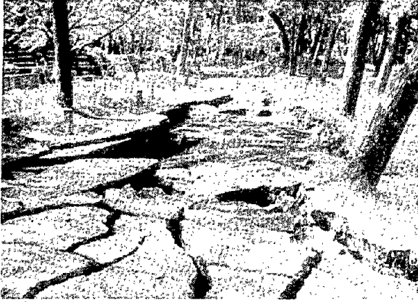
Photo 11 Ground Fissure in the Aoba-cho Graveyard
