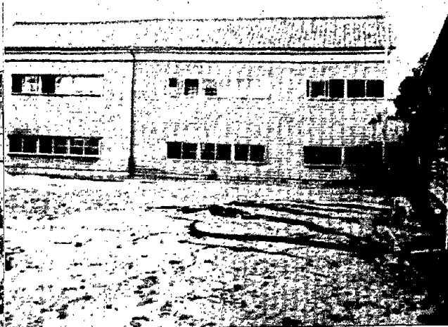
Photo 41 Ground Fissures in the School Playground
