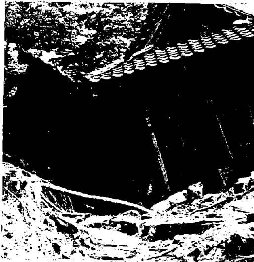
Photo 42 A Shrine Building Which Fell into a Ground Fissure
