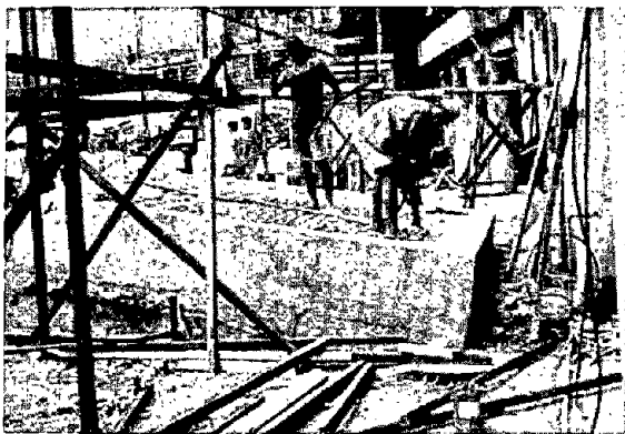
Photo 14. Floating of an underground septic tank at Luzon College.
