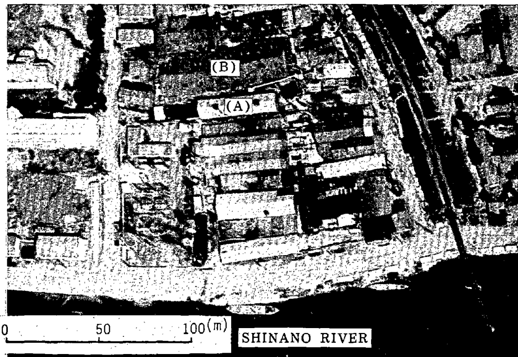
(b) After the Earthquake (1964)
