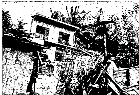
Photo 20. A house located at the left bank of the Pantal River. Since the foundation ground moved toward the river, the building tilted severely toward the river and its foundations failed.
