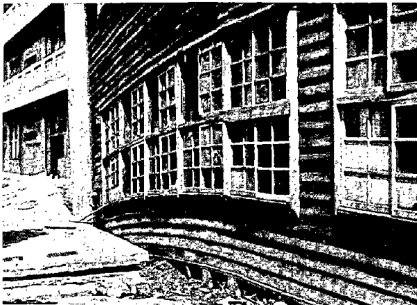
Photo 9 Distorted Building at Meikun High School
