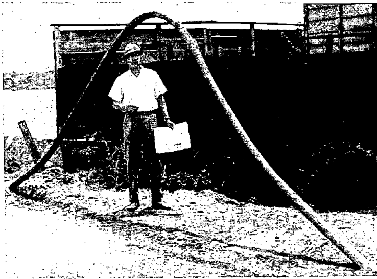
Photo 31 Buckling of a Buried Gas Pipe
