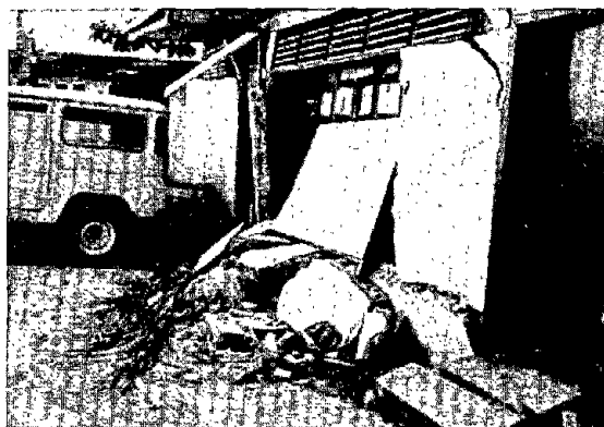
Photo 17. Damage to the exterior wall of the Philippine National Bank looking from the rear. The building was pulled by a lateral ground movement toward the Pantal River (to the left).
