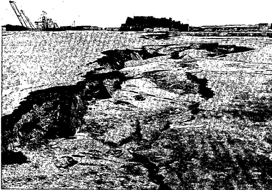
Photo 18 Ground Fissure at Gaiko Wharf
