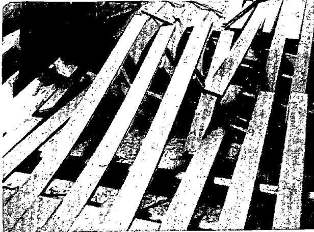
Photo 36 Broken Wooden Floor due to Ground Fissure
