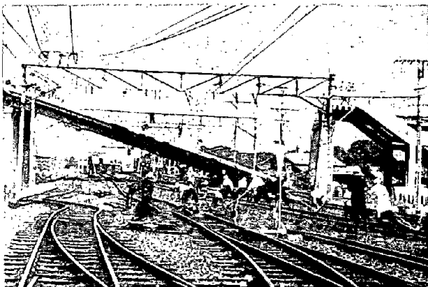
Photo 28 Collapse of the East Bridge over Railway (Point ④ in Figure 27(b)) 16
