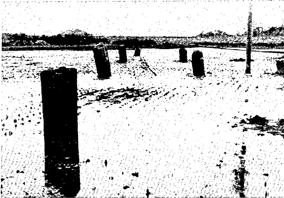
Figure 5 Seven Wooden Piers Which Buoyantly Rose about 1.5 m in a Rice Field during the Kanto Earthquake (Imperial Earthquake Investigation Committee, 1925) 11)
