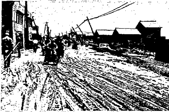
Photo 32 Route 7 after the Earthquake 18)
