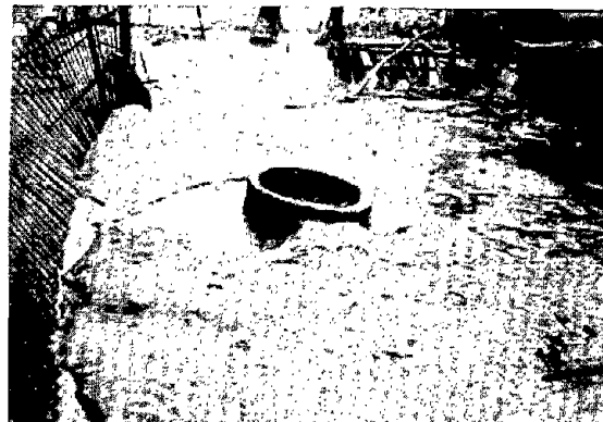
Photo 44. Well settled due to liquefaction. Sand nearby is thought to have boiled out. (Courtesy of Dr. M. Hakuno).
