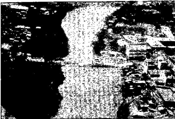
Photo 3. Damage near Magsaysay Bridge looking from upstream. Lateral spreading and submergence of the ground along both riverbanks are clearly seen (Courtesy of Dr. G. F. Wiczorek).
