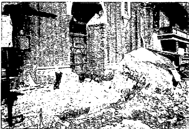
Photo 21. Collapse of tower of an old Catholic church facing Zamora Street, thought to have been caused by ground shaking (Courtesy of Mr. T. Nakajima).
