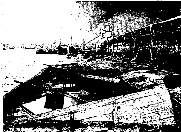
Photo 18 Damage to the Quay Wall at the Fishery Pier (Point ① in Figure 22(a))
