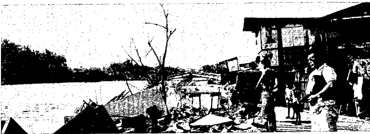
Photo 5. Riverbank behind Perez Market. The fence broke and collapsed into the river. Magsaysay Bridge is seen in the distance.
