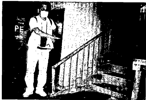
Photo 13. Damage of Luzon College due to liquefaction. The handrail was as high as the man's hand before the earthquake.
