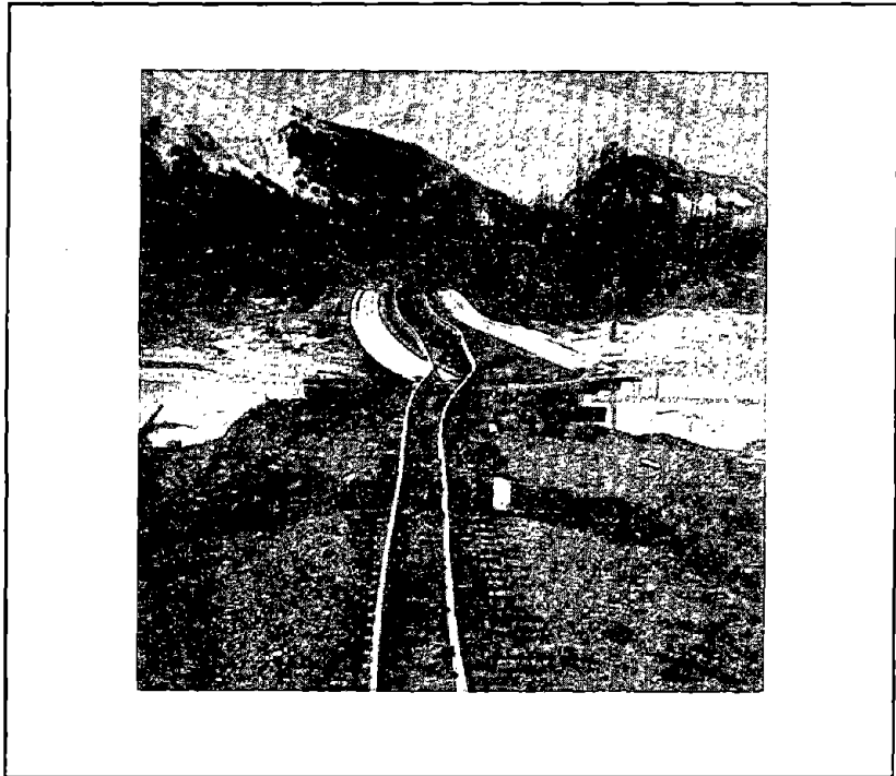
Figure 52 Damage to Bridge at Milepost 63.0 (looking south - from McCulloch and Bonilla, 1970).
