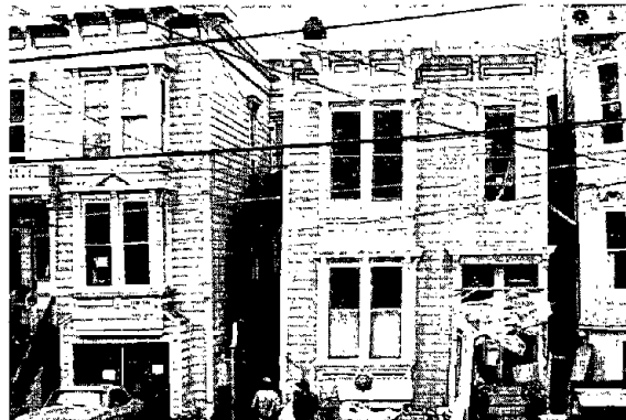
Photo d. Racking and Settlement of Houses on Shotwell St. Between 17th and 18th Sts. in 1989. These Houses are Directly Behind the Location of Houses in Photo c (photograph by T.D. O'Rourke)
