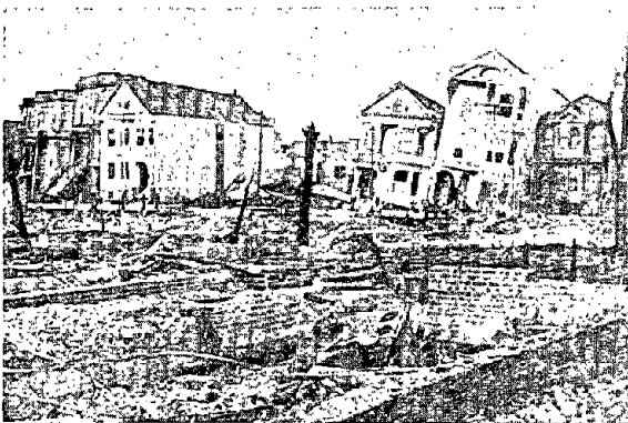
Photo c. Racking and Settlement of Houses on South Van Ness Between 17th and 18th Sts. in 1906 [after Lawson, et al., 1908]
