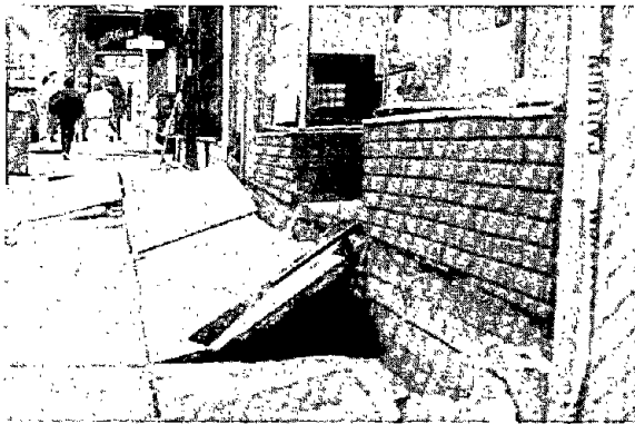
Photo a. Differential Movement of 100 to 300 mm Adjacent to Building at Corner of 7th St. and Natoma St. (photograph by T.D. O'Rourke)
