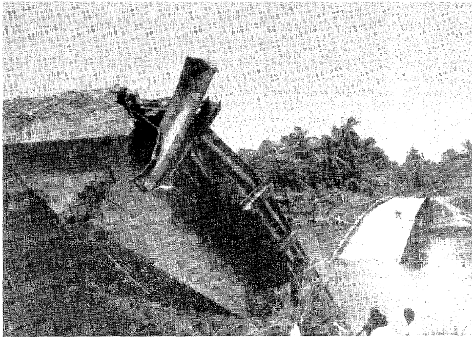
Rio Vizcaya Bridge: Liquefaction Failure During 1991 Costa Rica Earthquake (Ref. 7, fig. 6-21, pg. 74, reprinted by permission of Earthquake Engineering Research Institute).
