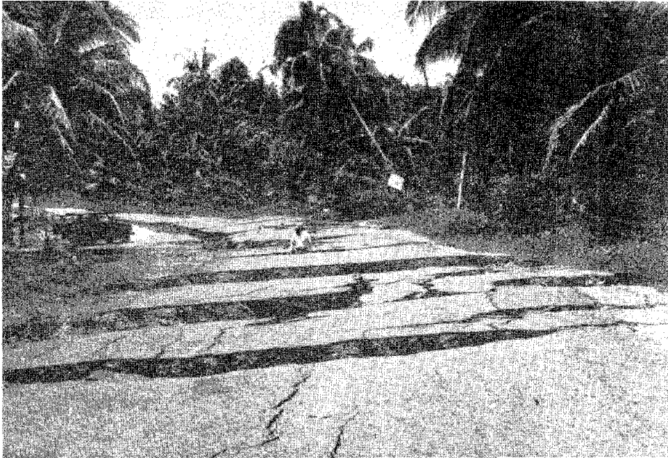
Rio Vizcaya Bridge: Fissures in the South Roadway Approach in 1991 Costa Rica Earthquake (Ref. 7, fig. 6-25, pg. 76, reprinted by permission of Earthquake Engineering Research Institute).
