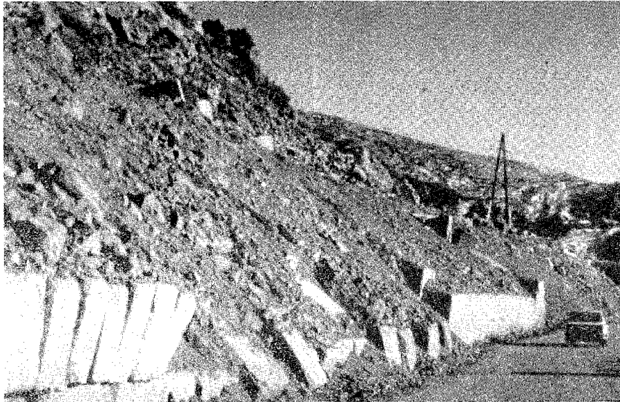
Failed Concrete Retaining Walls Near Spitak in 1988 Armenia Earthquake (Ref. 4, fig. 5.13, pg. 65, reprinted by permission of Earthquake Engineering Research Institute).
