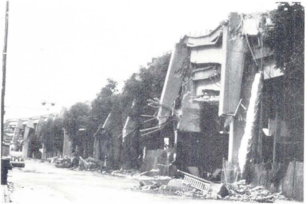
Fig. 1.12 Collapse of the I-880 Cypress St. Viaduct.
