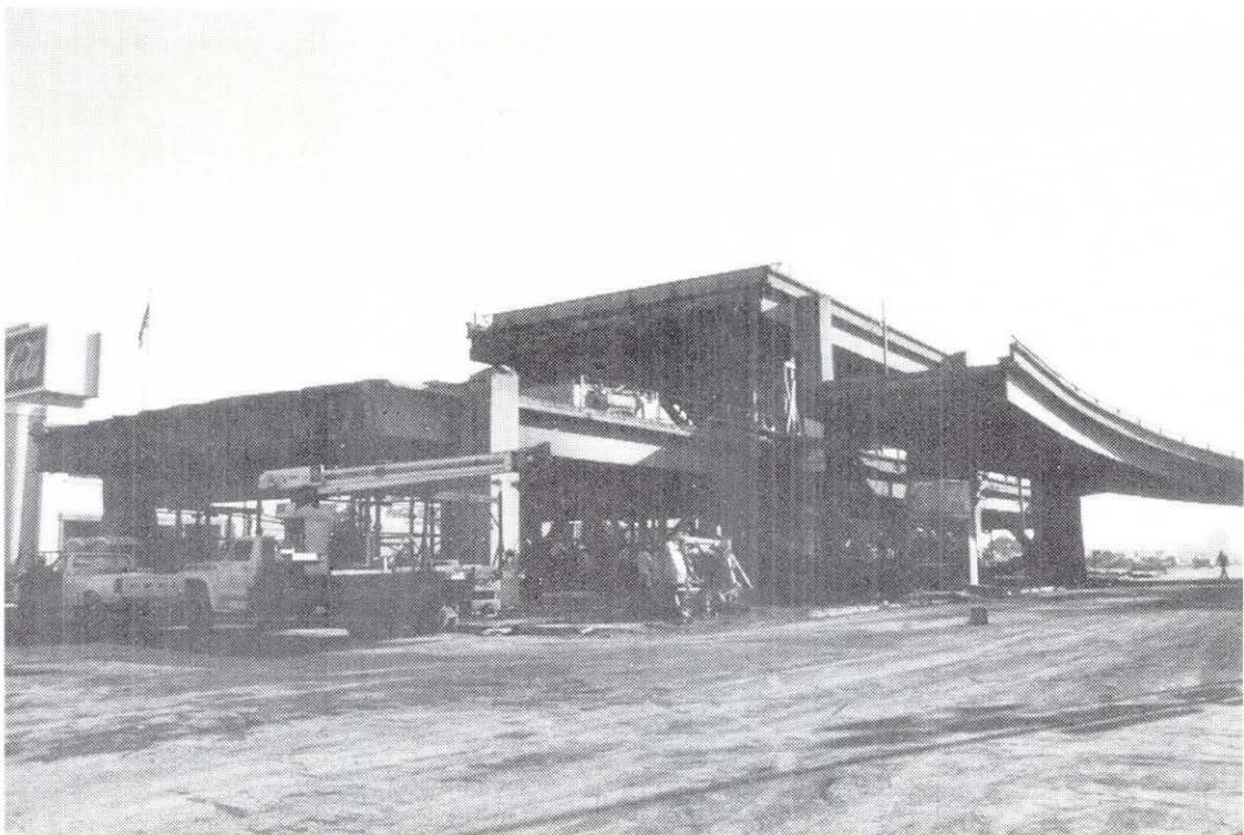
Fig. 2.3 Ground level photo showing Bents 47-48.
