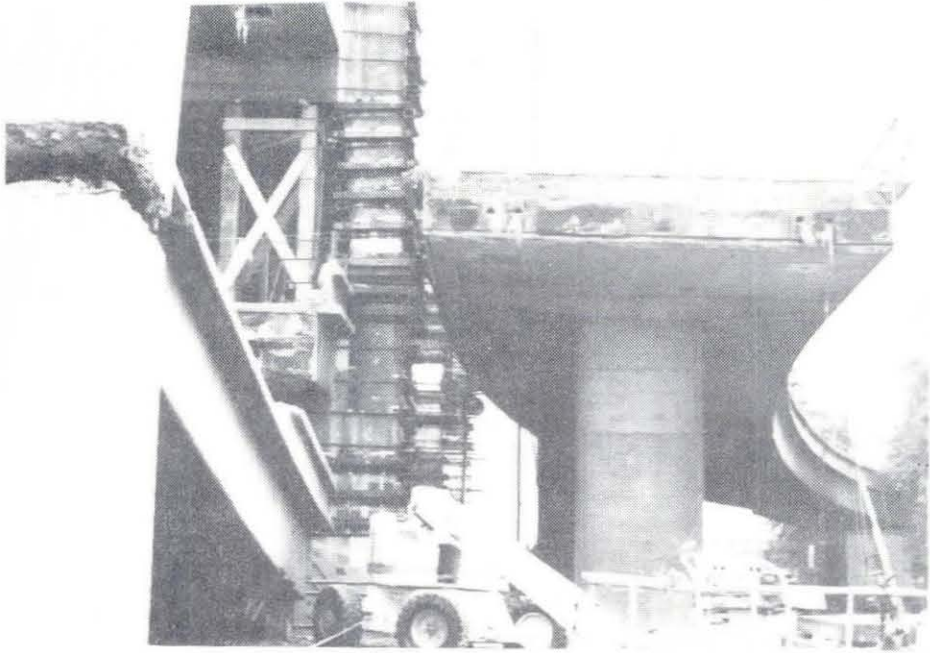
Fig. 2.4 Ground level photo showing separation of test specimen from off-ramp.
