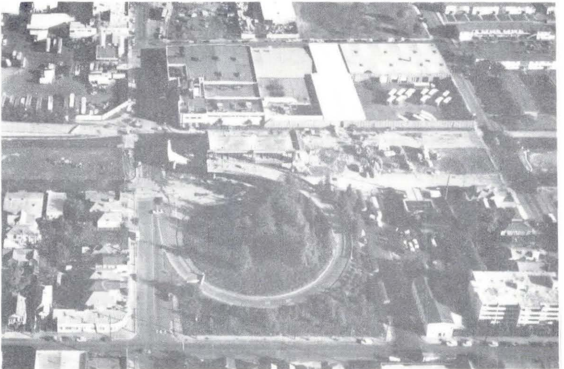
Fig. 2.5 Aerial photo showing test specimen and adjacent off-ramp.
