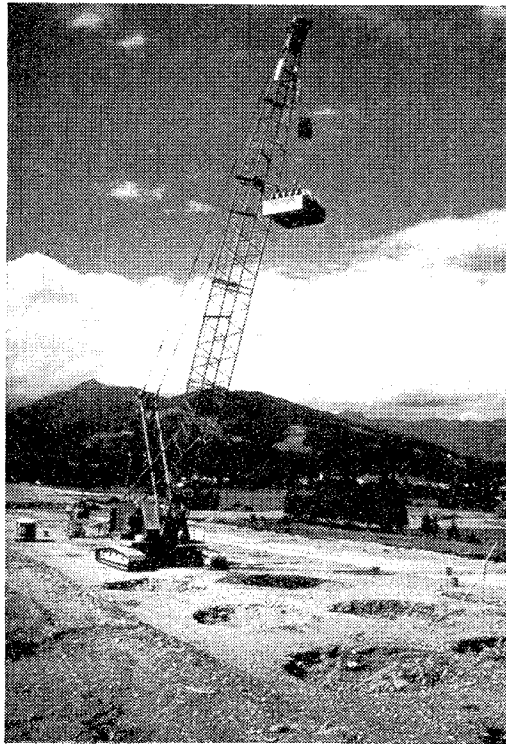
Fig. 3 Illustration of Dynamic Deep Compaction
