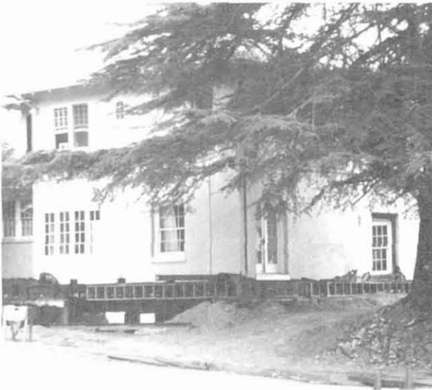
Figure 4.2.6. House jacked up for foundation repairs.
