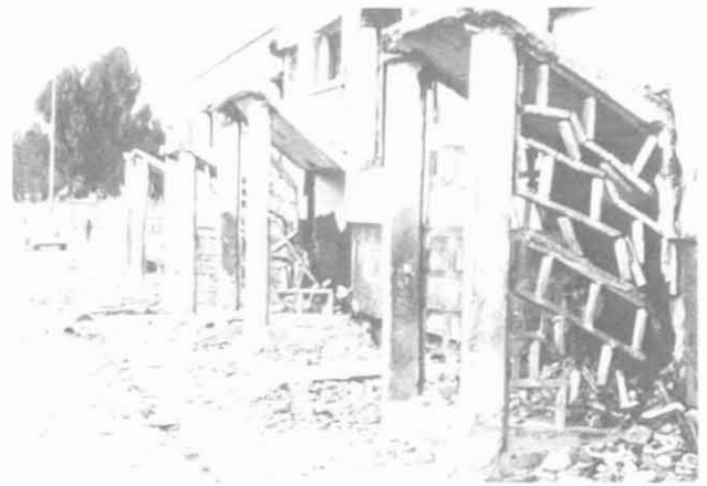
Figure 3.4.3. Building damage in El Asnam.
