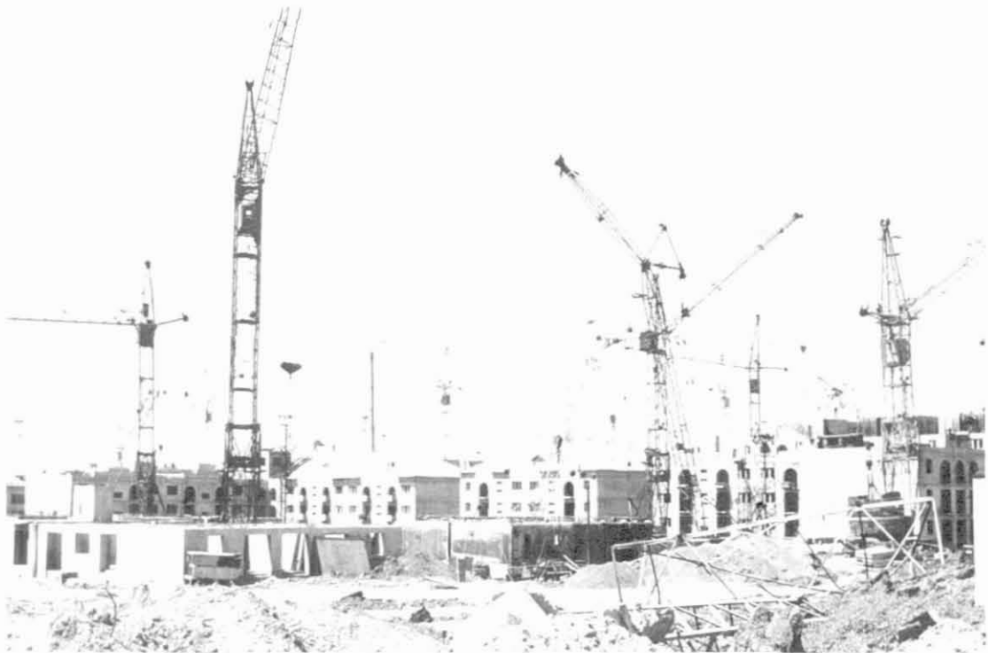
Figure 3.6.10. Construction site with cranes.
