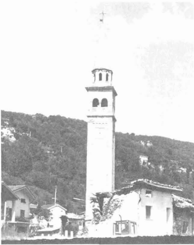
Figures 3.3.2. Damaged church in Forgaria with campanile amazingly still standing. Photo courtesy of the Earthquake Engineering Research Institute (EERI).
