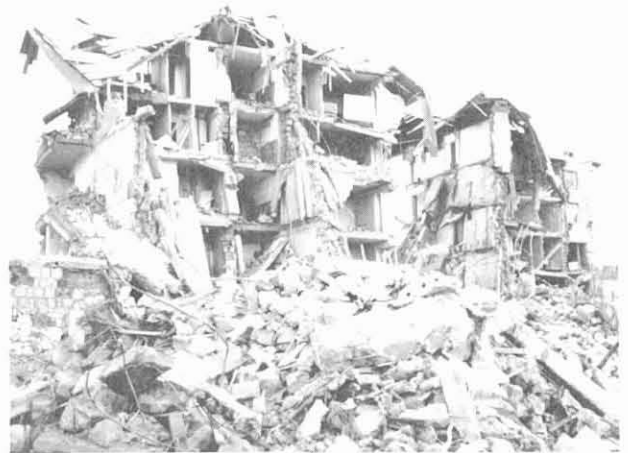
Figure 3.6.4 Destroyed masonry building in Leninakan. Photo courtesy of the Earthquake Engineering Research Institute.
