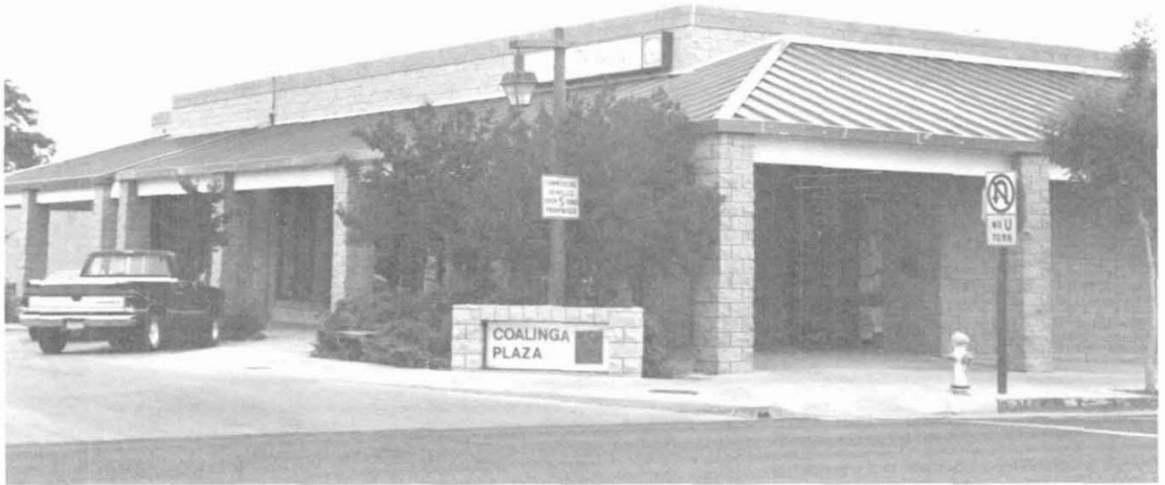
Figure 4.1.6. EDA building in downtown Coalinga, May 1990.
