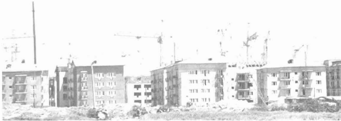
Figure 3.6.11. New housing under construction near Leninakan.
