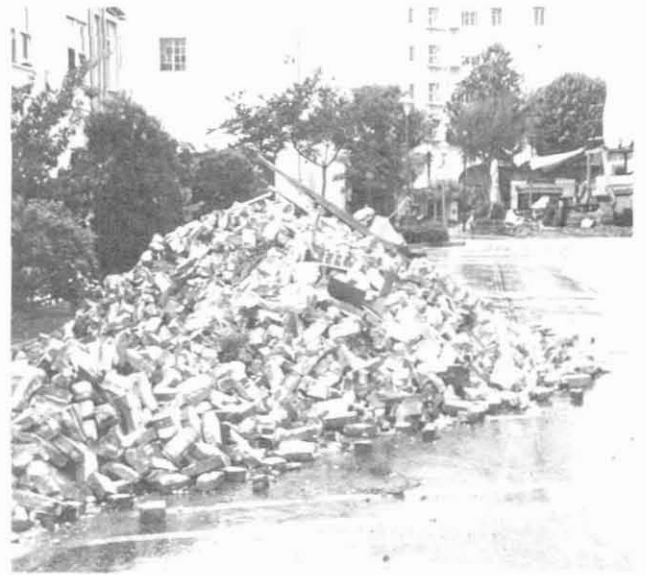
Figure 4.2.4. Pile of used bricks for use in rebuilding.
