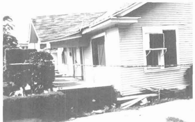
Figure 4.2.2. Damaged single family house in north Whittier.
