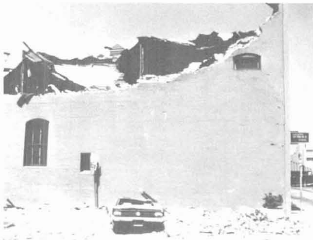
Figure 4.2.1. Damaged unreinforced masonry building in Uptown commercial area.
