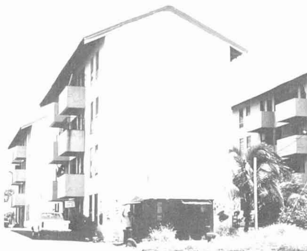
Figure 3.2.12. New apartment building.
