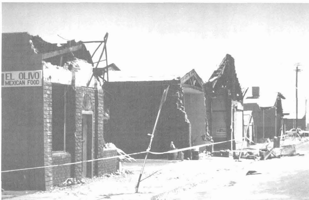
Figure 4.1.1. Destroyed unreinforced masonry buildings in downtown Coalinga.
