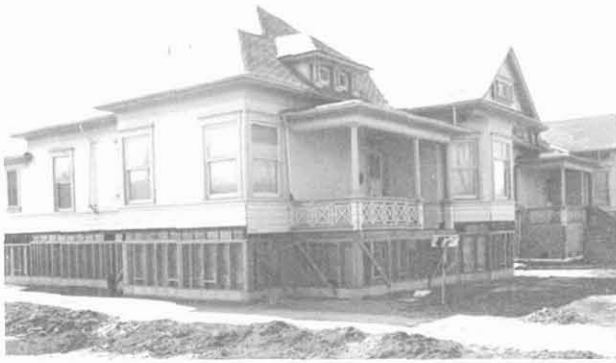
Figure 4.3.11 Single family home being repaired.
