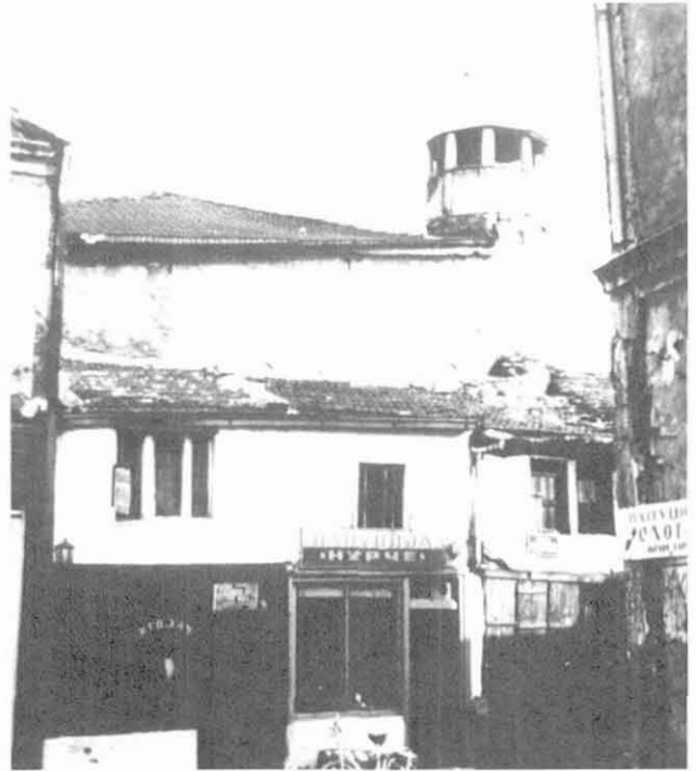
Figure 3.1.10. Building in historic area of Skopje, waiting to be rehabilitated and strengthened.
