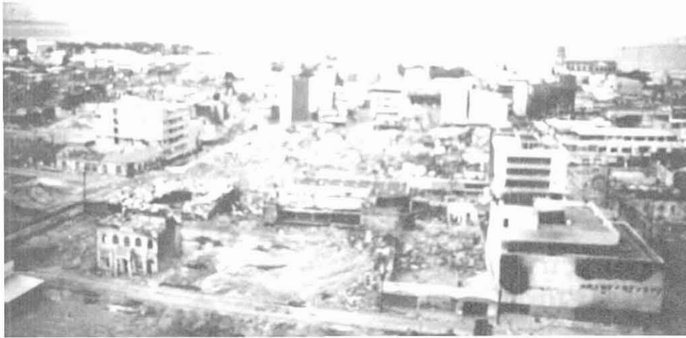
Figure 3.2.2. Earthquake destruction in central Managua.
