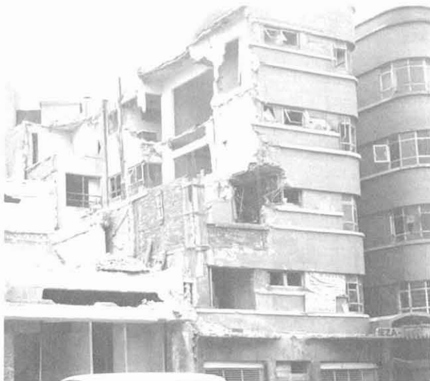
Figure 3.5.2. Damage in central Mexico City, photographed in February 1986 by William Spangle and Associates.
