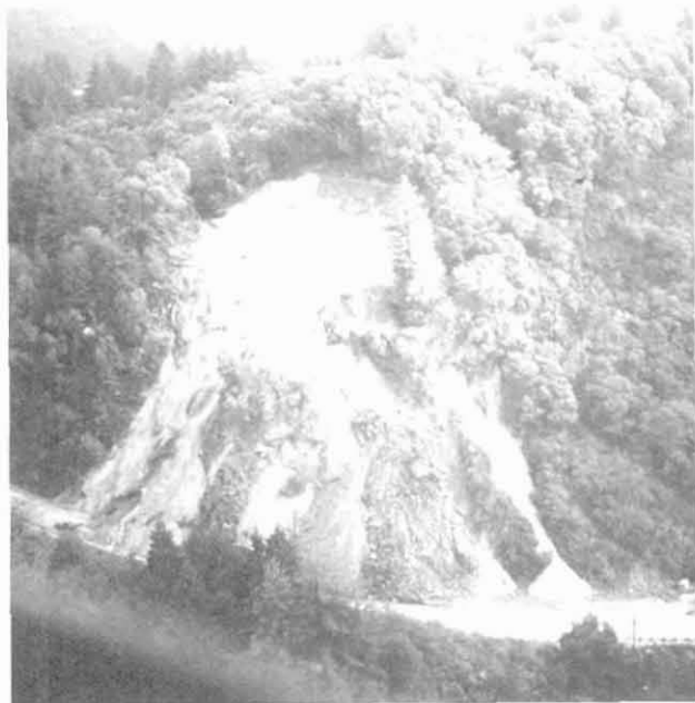
Figure 4.3.2. Landslide in Santa Cruz Mountains on Highway 17. Photo courtesy of William Cotton & Associates.
