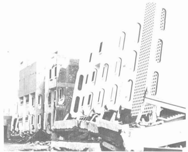
Figure 3.4.4. Damage to buildings supported by slender columns.
