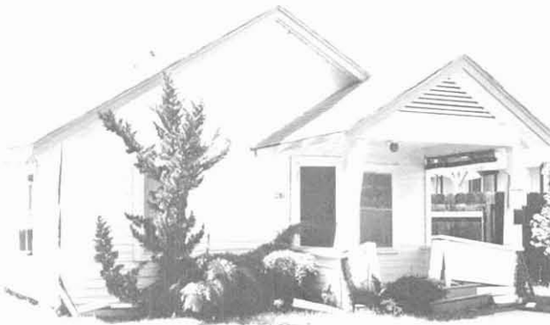
Figure 4.1.2. Damaged single family house.
